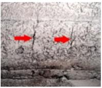
Figure 2. Cracks in the steam drum to dish end weld
