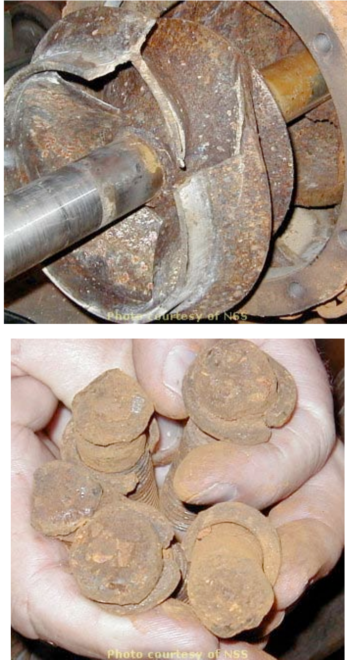
Figure 7.19 Impeller and bowl bolts from the tower water pump evaluated by PSAT in Figure 7.18
