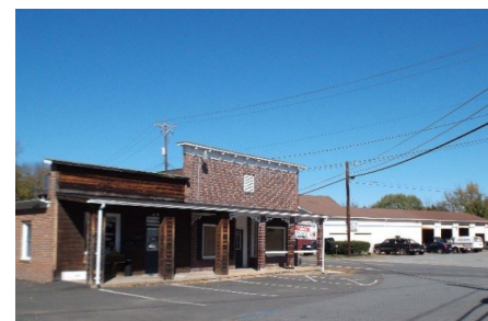
Historic Commercial Development at the Intersection of Old Catlett & Elk Run Rd
