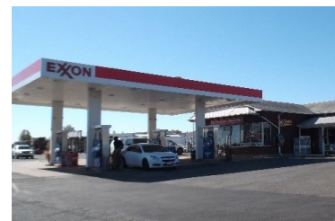
Exxon Station at Catlett Market and Deli Complex
