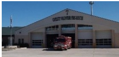
Catlett Volunteer Fire-Rescue Station
