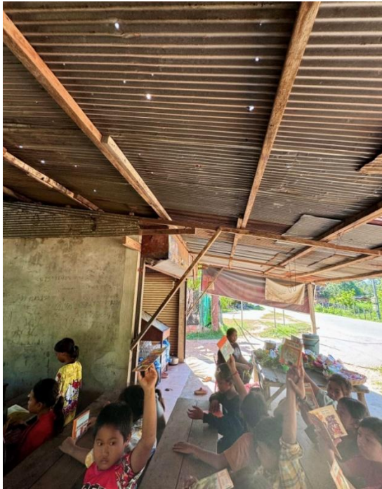
Check out the holes in the roof
