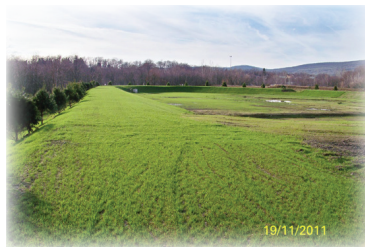
Reclamation of Misty Ridge in Old Forge
