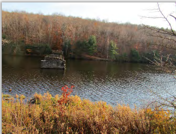
Elmhurst Reservoir bridge site along E&WV RR and PA Route 590
