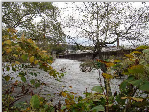
Looking upstream from confluence with the Lackawanna River in South Scranton
