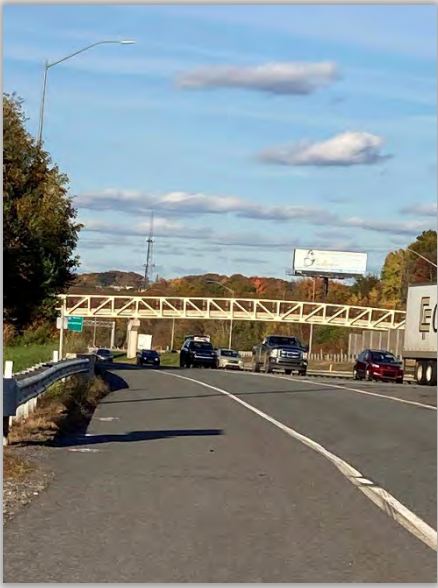
Pedestrian Bridge over I-81 at Avoca
