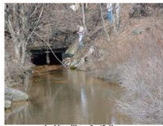
1. Vanding Outfall Vanding
