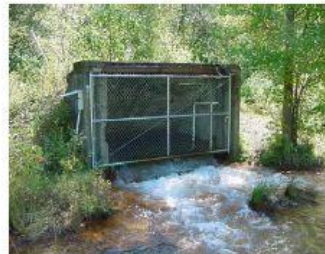
7. Gravity Slope Outfall Archbald
