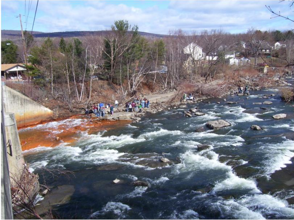
Figure 1-2 The Old Forge Borehole entering the Lackawanna River's western bank.
