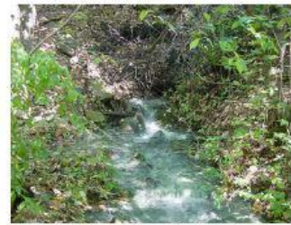
5. Dana Tunnel Outfall Archbald
