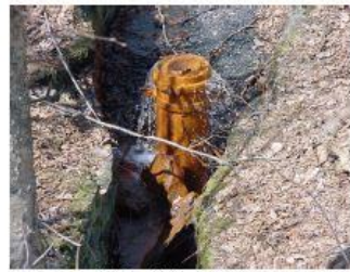
2. Standpipe Outfall Vanding
