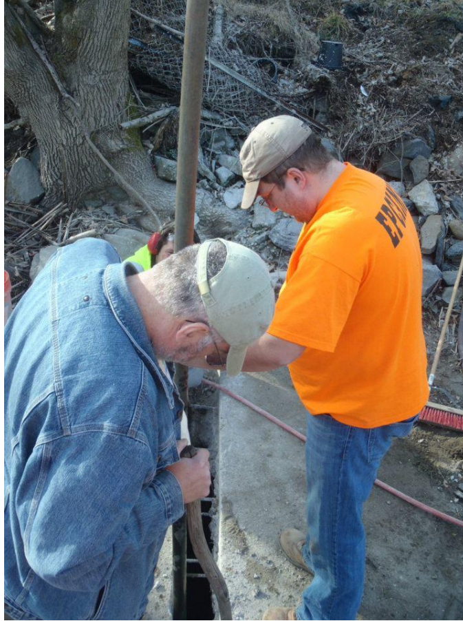
Figure 6-4 Study team decides how to take flow measurements and install transducer in concrete cap opening.
