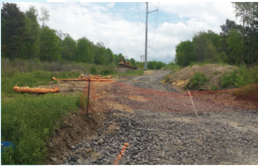
PPL line along Quinton Road, Scott Twp.
