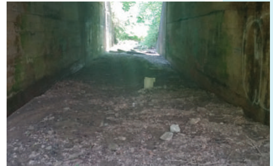
Tunnel under active rail road
