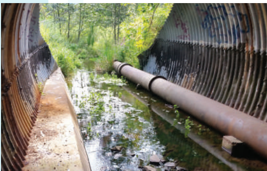
Sanitary line under Leggett's Creek culvert
