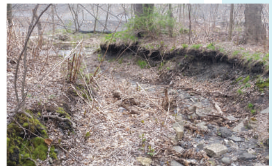
Create step-pool system in failed ditch
