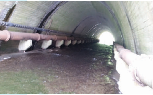
The Notch Connector trail can utilize culvert under expressway
