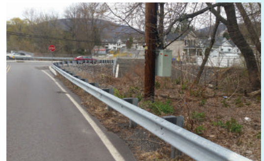
Bioswale location along top-of-bank
