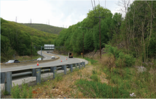
Room to enter Notch along ramp
