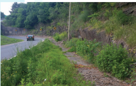
Existing walkway near Oak Street ramp
