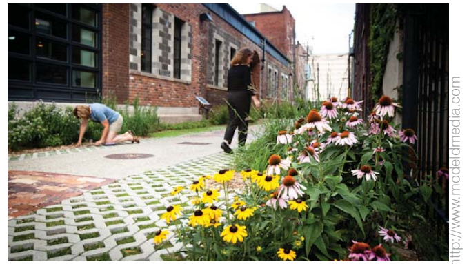
Example of a green alley using permeable pavers and vegetation.
