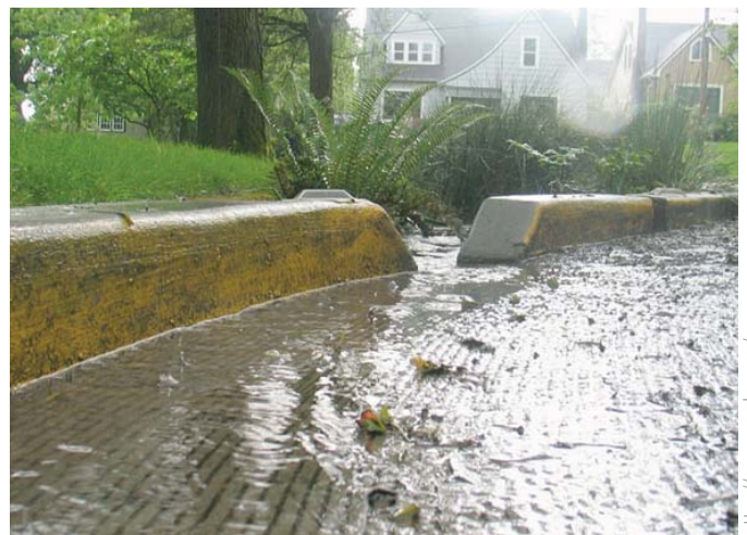
Water flowing through a curb cut into a bumpout.
