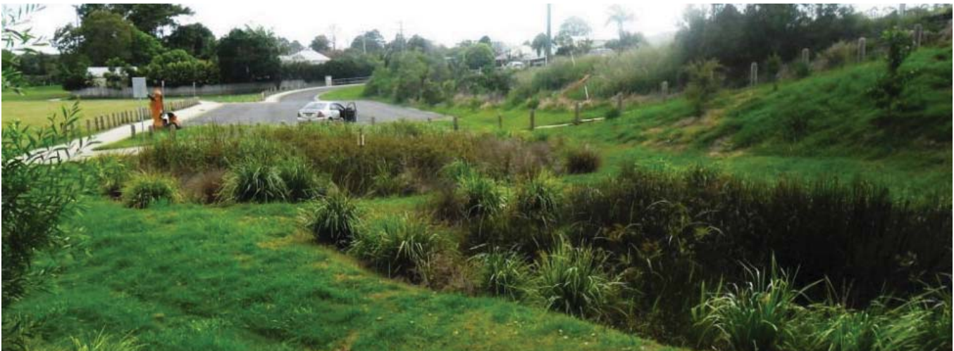
An example of a constructed wetland that filters runoff from an adjacent street.
