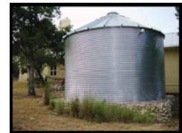
Above ground cistern.
