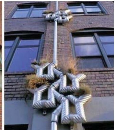
Incorporating the planter into the downspout is another option when room is limited.
