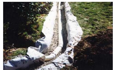
A french drain before it is covered with dirt.
