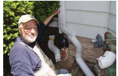
Bernie McGurl, LRCA, completes a downspout disconnect demonstration project.
