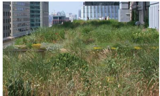
Data collected from Chicago's City Hall's green roof indicate that the roof not only reduces stormwater runoff by 50 percent, but significantly reduces energy use and saves the City approximately $5,500 annually on heating and cooling expenses 22
