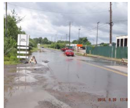
Flooding along Boulevard Ave. near I-81 swale
