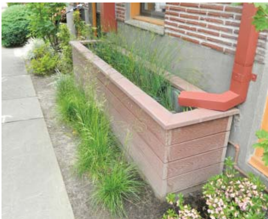
A downspout planter can be located next to a building.
