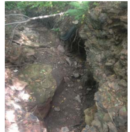
Philo Creek: evidence of erosion
