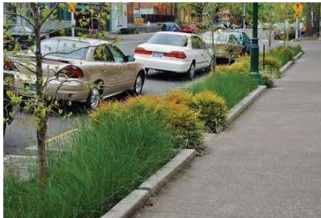
Unused area on sidewalk converted into vegetated swale.
