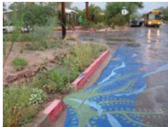
A curb cut that allows water to enter a site. The painted pavement makes the use of the curb cut more obvious to the public.
