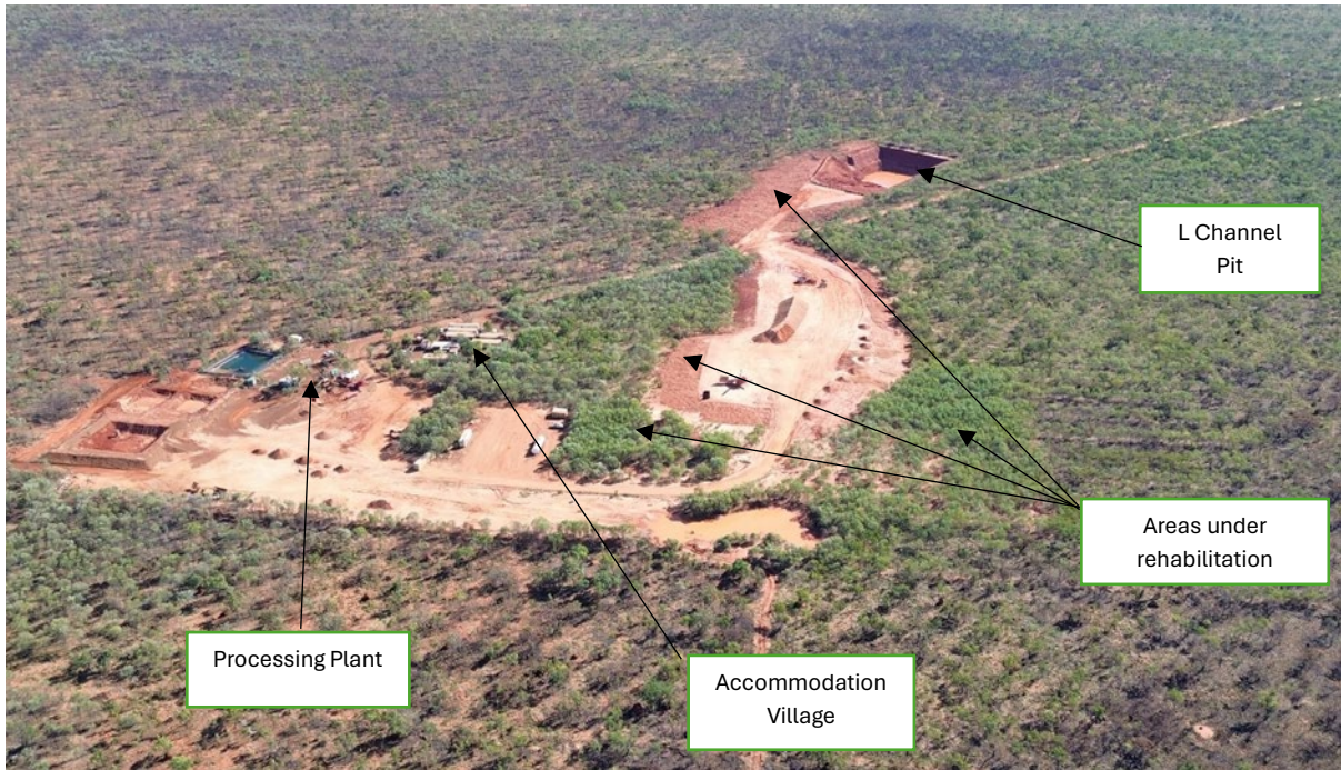
Figure 6: Aerial view of the Ellendale Mine operations area & the L Channel alluvial pit, June 2023.
