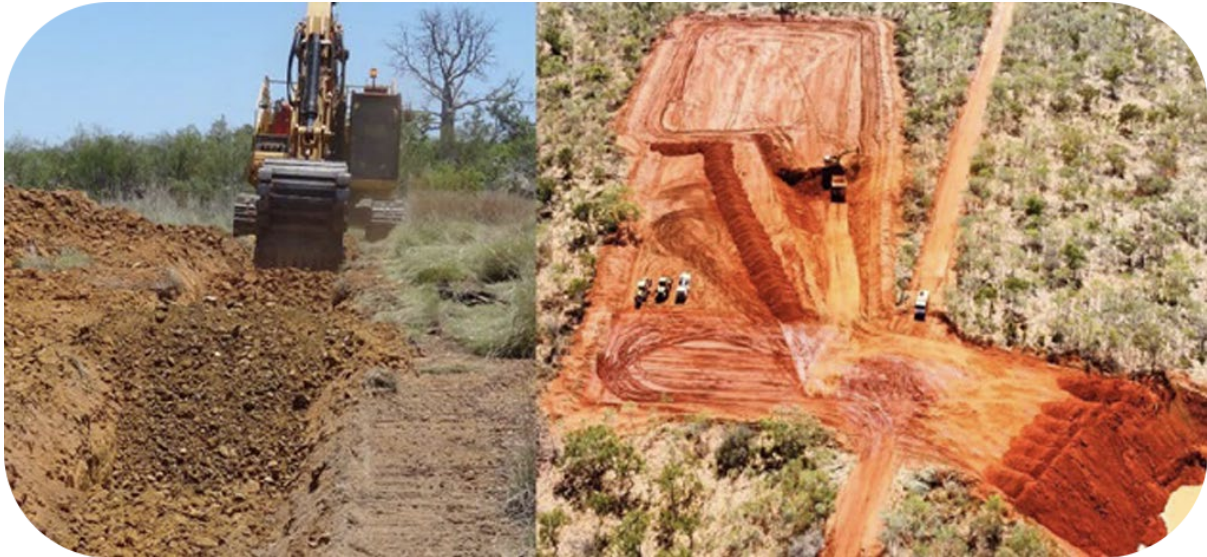
Figure 4: Bulk sampling of shallow gravel. Figure 5: Mining & backfilling in the L Channel.
