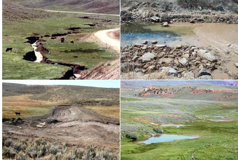
Top-left: Eroding stream banks along Rees Creek above the sediment ponds.
