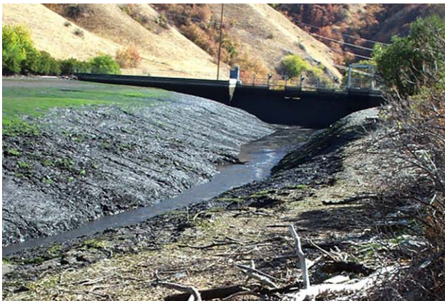
Left: Upstream view of sediment behind First Dam when it was drawn down for repair. Right: Downstream view of First Dam after upgrade. (Photos courtesy of Utah Water Research Laboratory.)
