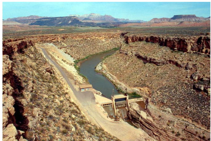
Quail Creek Diversion Dam on the Virgin River near Hurricane Utah. (Photo by Ron Ollis).
