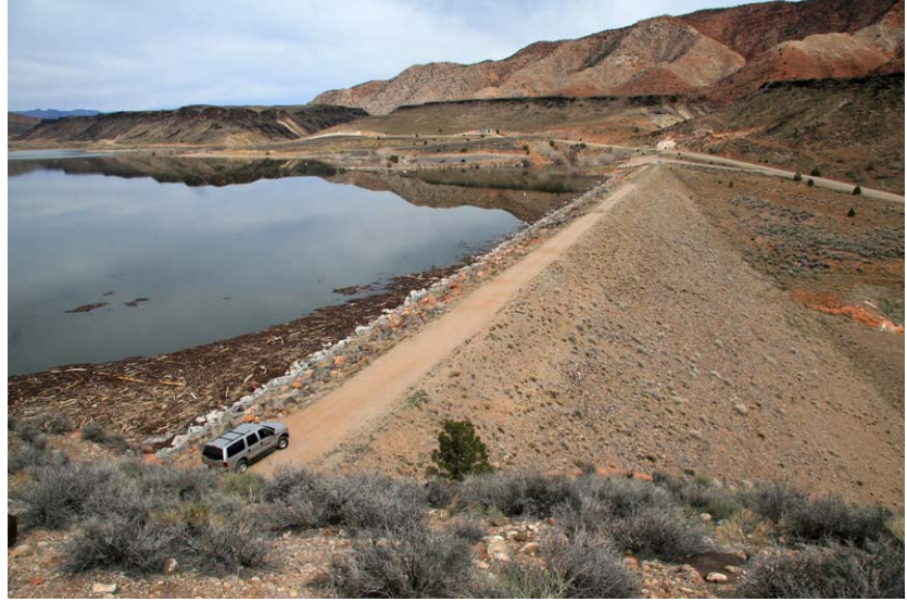
Gunlock Reservoir. Debris, left over from flooding, can be seen in lower left-hand corner. Debris, such as this, covered the entire surface of the reservoir after the large flooding events of 2005 and 2007.
