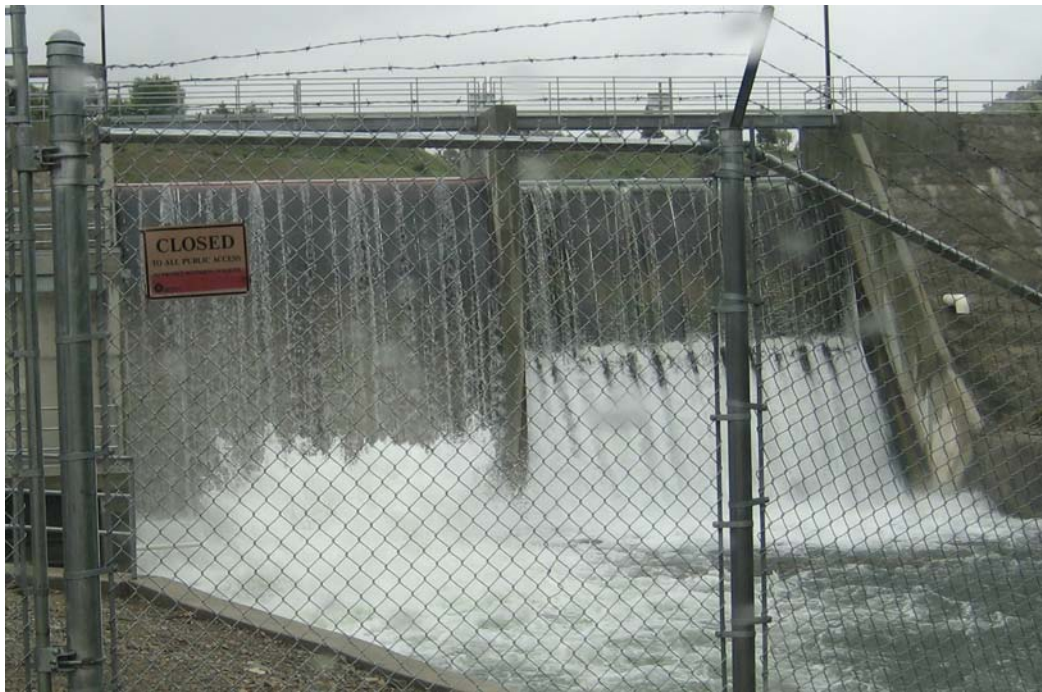
Figure 6: Use of Spillway Releases to Aerate Discharge from the Low-Level Outlets on First Dam (shown on the spillway on the left)
