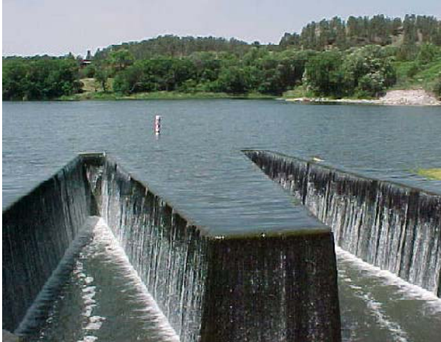
Labyrinth spillway design at Valentine Mill Pond. (Photo by John Bender, Nebraska Department of Environmental Quality.)
