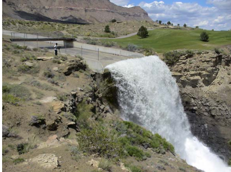
Clear water spilling out of Millsite Reservoir.
