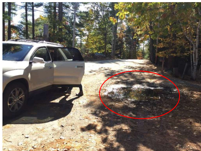
Photo 2: View at boat ramp entrance where runoff ponds along the southwestern edge of pavement.
