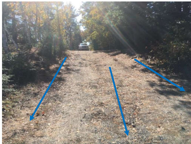
Photo 1: View up the boat ramp with erosion along edges and down the approximate centerline.
