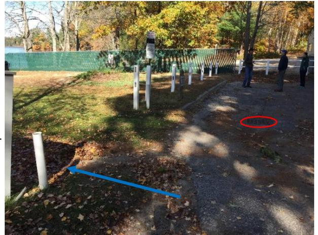
**Photo 5:** View northeast toward Town Beach. Stormwater bypasses the existing catch basins at the curb break in the foreground.
