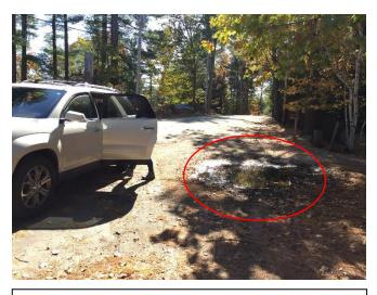
**Photo 2:** View at boat ramp entrance where runoff ponds along the southwestern edge of pavement.
