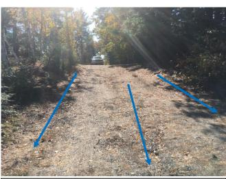
**Photo 1:** View up the boat ramp with erosion along edges and down the approximate centerline.
