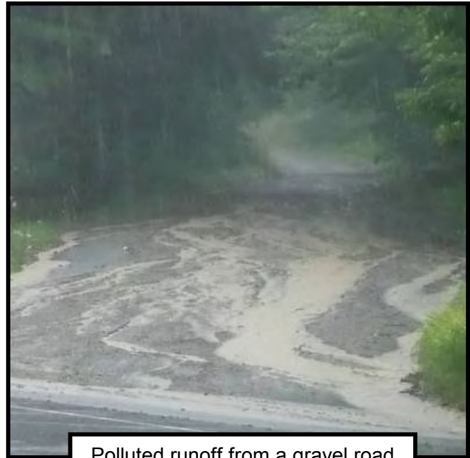
Polluted runoff from a gravel road
