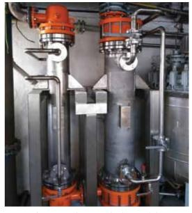
≈ Two exchangers (condensers) with Silicon Carbide (SiC) tubes have replaced graphite exchangers at an Italian API company.
