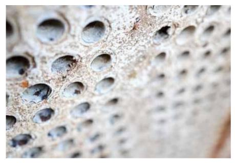
≈ Heat exchanger opened for inspection.
