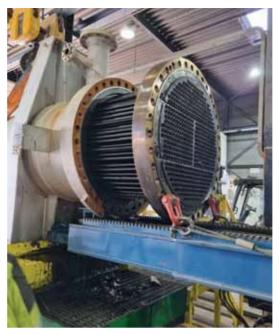
≈ Total Cleaning includes complete removal of heat exchanger and its shell for cleaning. Once the unit is properly maintenanced, it's returned to the customer ready for immediate installation and use.
