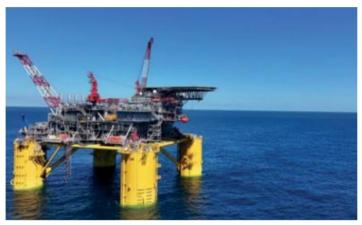
Shell's Whale platform, the company's second deepwater project in the Gulf of Mexico, has successfully launched with a simplified design based on the Vito project. The platform features a 99% replicated hull and 80% replicated topsides from Vito, which began production in 2023. Whale, weighing 25,000 tonnes, is one-third the size of Shell's Appomattox platform and designed to produce 100,000 barrels of oil equivalent per day. It also incorporates energyefficient gas turbines, reducing
