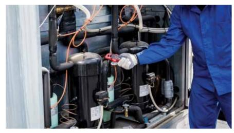
≈ The technician checking power lines of the heat exchanger with current clamps.
