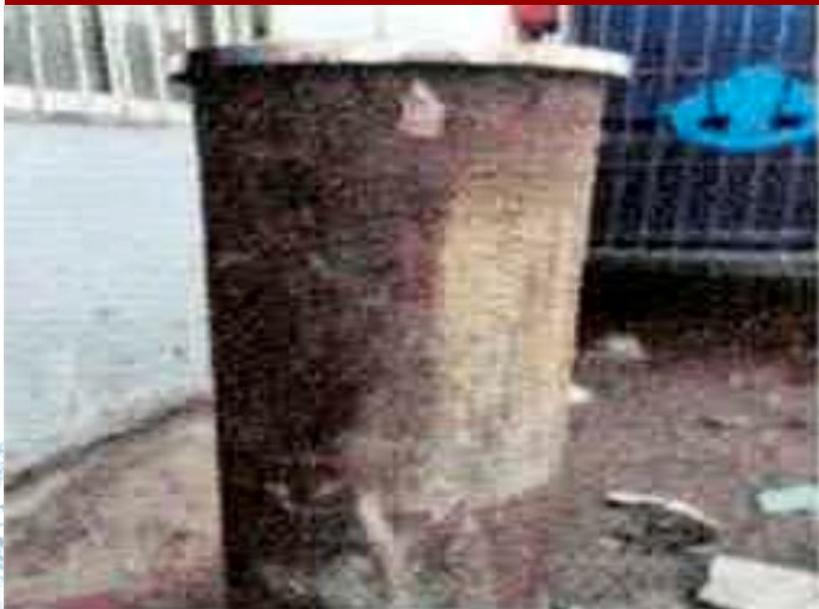
Salt crystal formation on central water pump filter in coal mine
