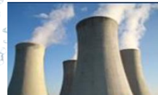
Electrical Power Industry
