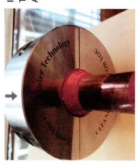
Installing the NAWT Collar at the front of the main water inlet pipe, The iron and calcium ions in the incoming water can be treated At the same time.
