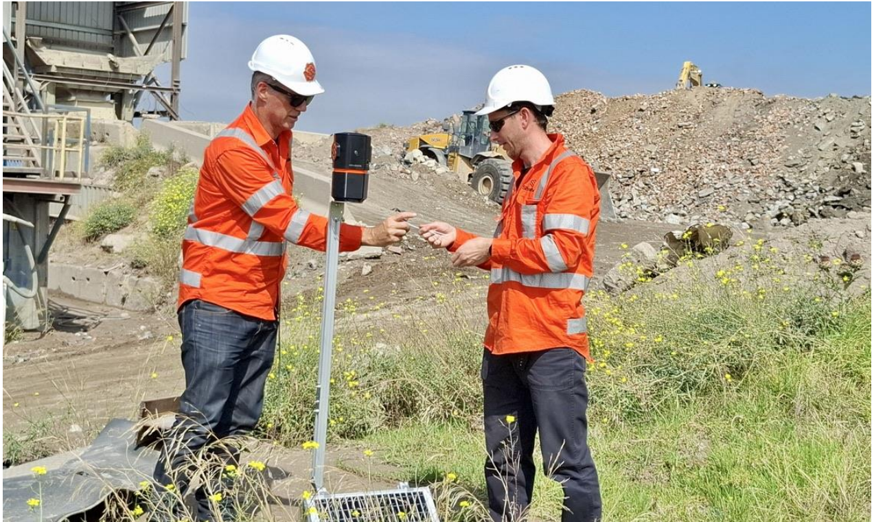
Pic: SiteHive personnel installing new sensors at City Circle Group in 2026.
