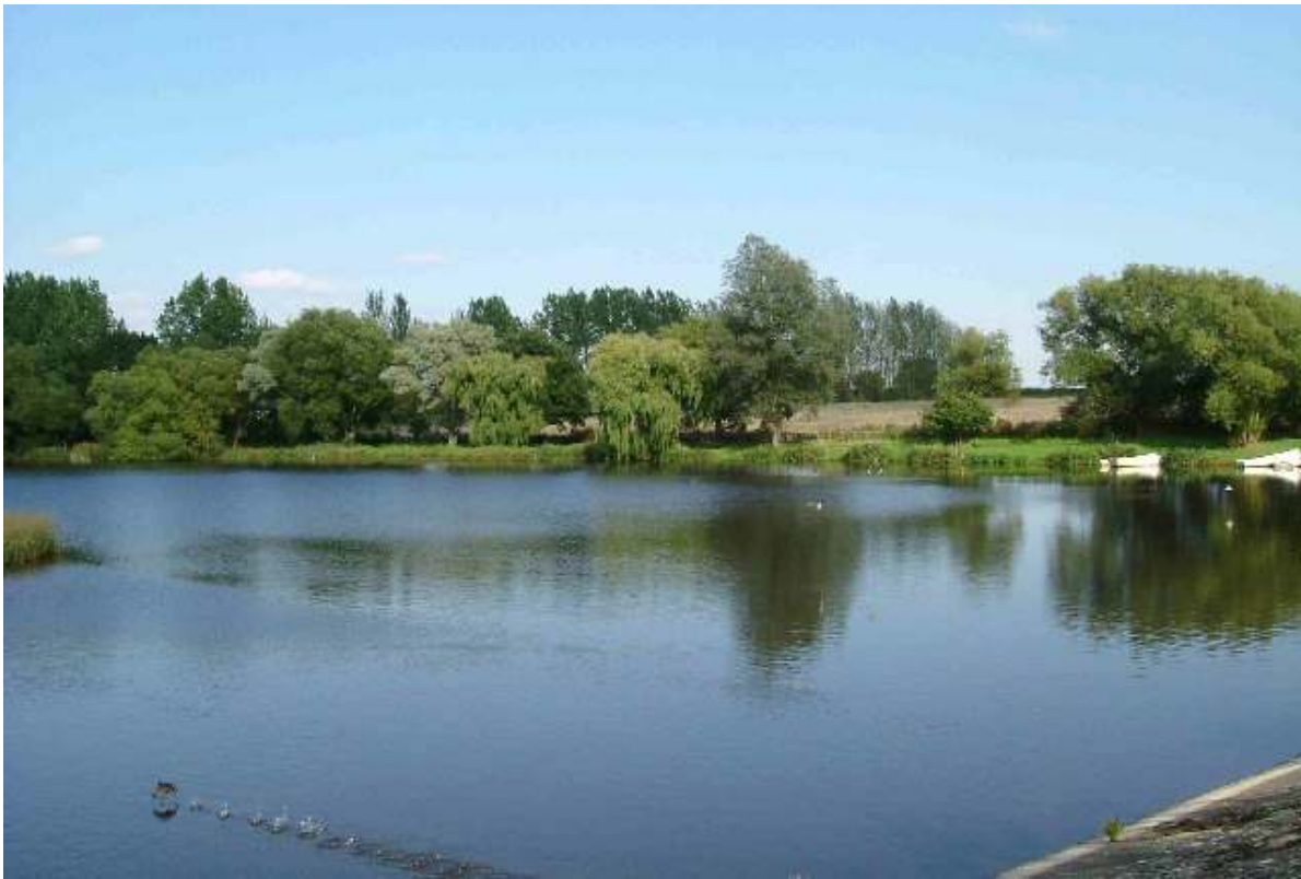
Fig. 16. Ardleigh Reservoir from Wick Lane
