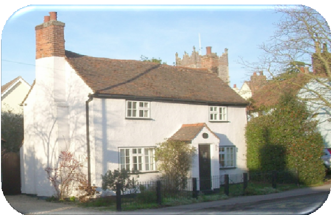
An example of a rendered, timber-framed building
