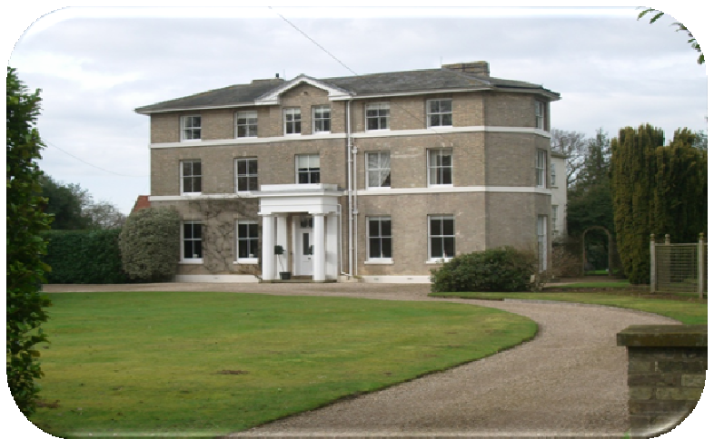
Elegant facade with a low-pitch slate roof
