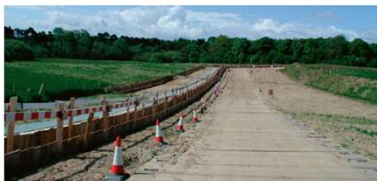
A cable is laid during construction with a single cable trench open
