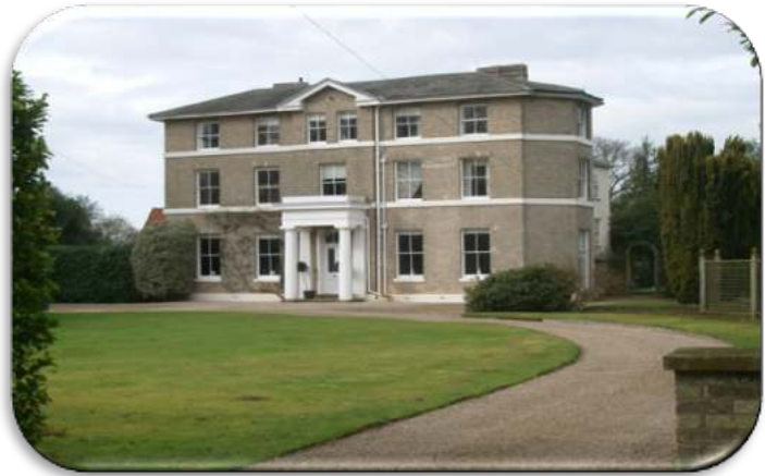
Impressive facade, with low-pitched slate roof emblematic of the Victorian era
