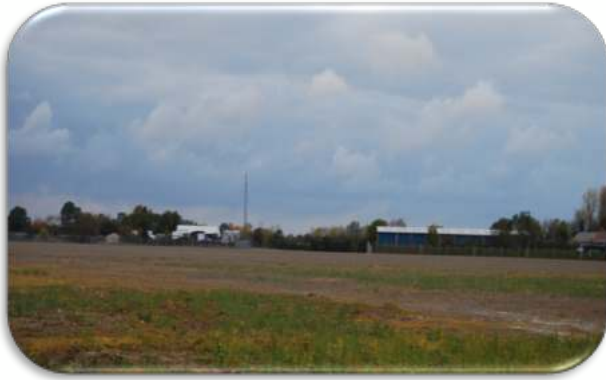
Industrial buildings on Old Ipswich Road as seen from Wick Lane
