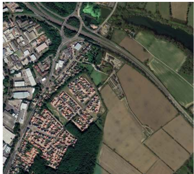
Aerial view of the Ipswich Road (including Plains Farm) area c. 2021
