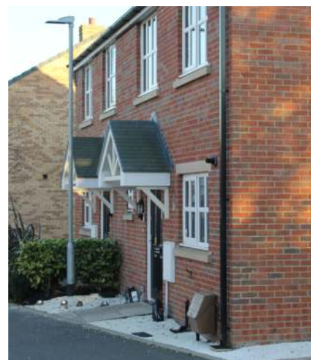
Contemporary dwellings at Ingrams Piece - the porches appear tacked-on rather than an integral part of the design
