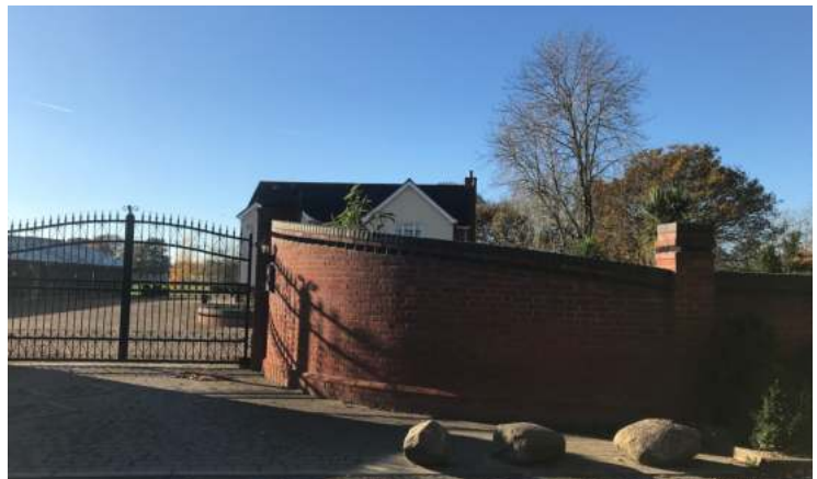
Inappropriate boundary treatments in new housing on Home Farm Lane
