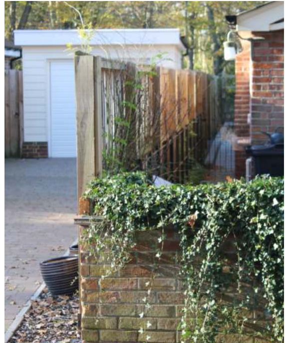
Traditional iron railing obscured by insensitive close-boarded fencing
