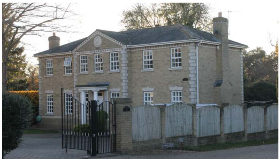
Close-boarded fencing is obtrusive and incongruent in the context of Ardleigh
