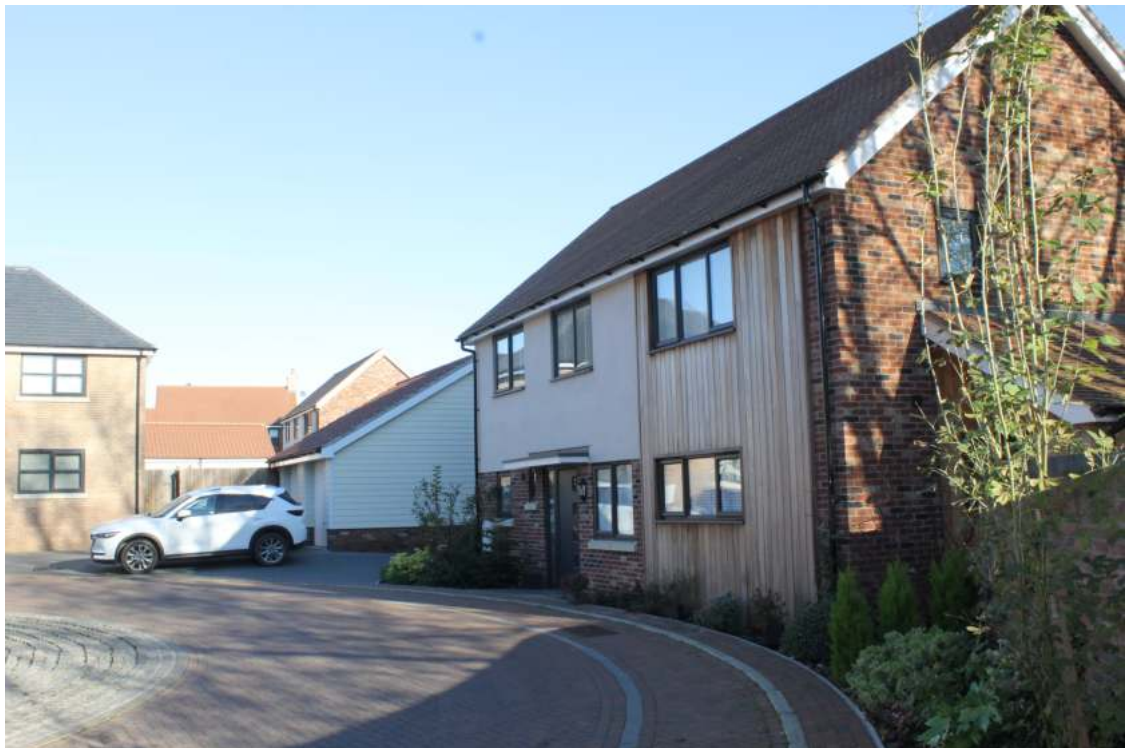
The new houses employ a mix of traditional and more contemporary local materials with great success
