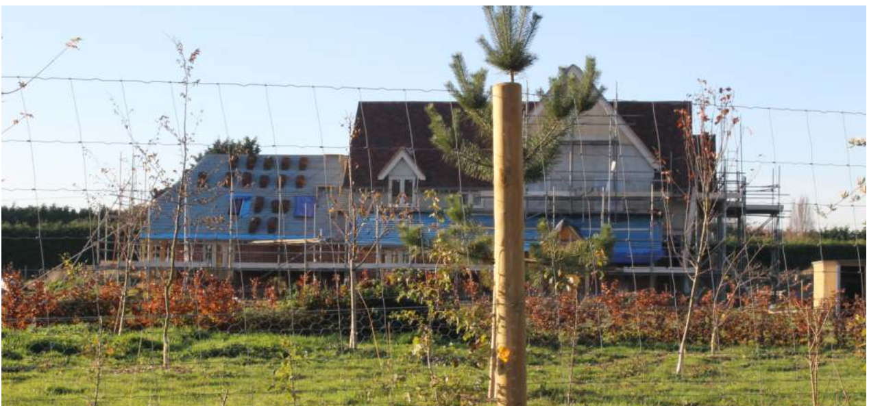
Stage of construction c. November 2021
