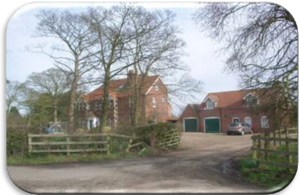
Badley Hall, Little Bromley Road
