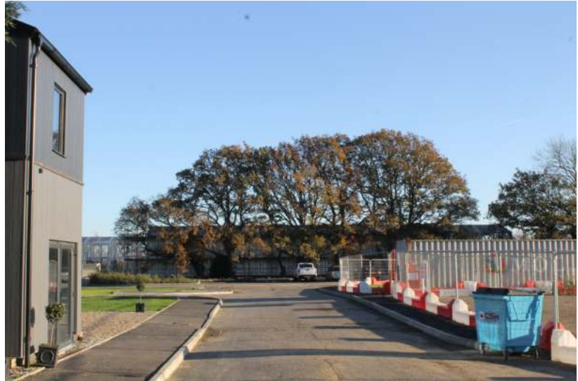
Construction underway at Crown Business Park, Old Ipswich Road
