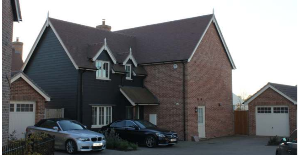
Dormer windows appear “cramped in” and relate poorly to the roof and building form
