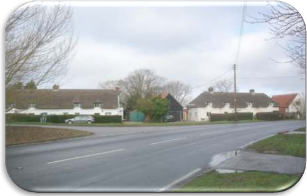
Thatched cottage, Dead Lane (Grade II listed) featuring thatched roof with eye-brow dormers
