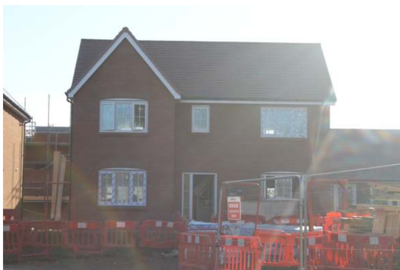
1 of the 145 dwellings under construction on Bromley Road
