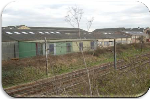
Industrial buildings in Home Farm Lane
