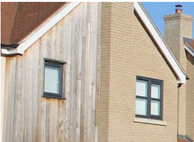
Metal windows add considerably to the design quality of this modern build
