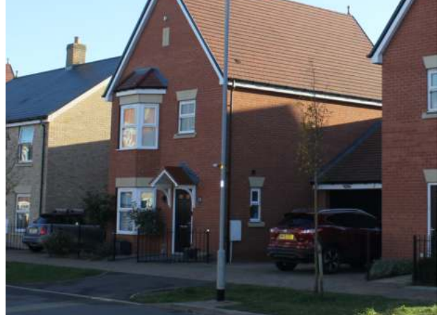
Despite this scheme having been approved and constructed in the late 2010s, its garages are built too small for modern cars, leading to unsatisfactory parking arrangements
