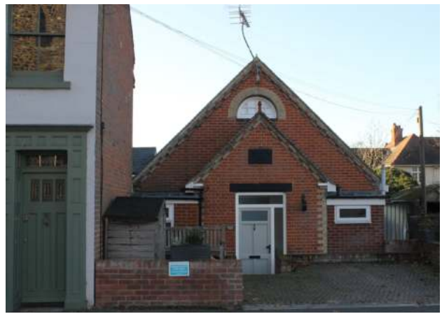
UPVC windows are an intrusive addition to this traditionally-styled property
