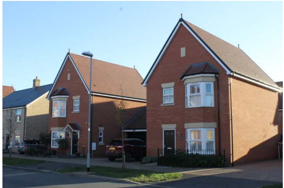
Garages built too small for modern vehicles
