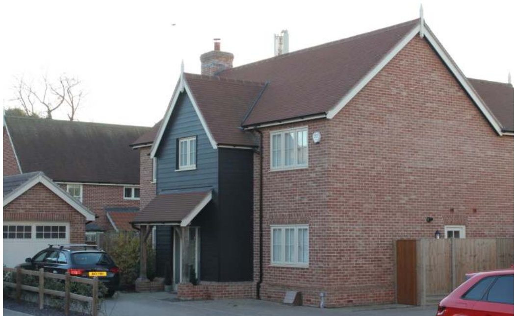
Expansive and predominantly blank elevations are symptomatic of poor and ill-thought-out design
