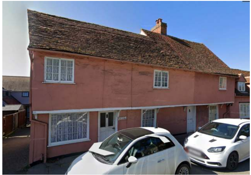
16th Century Tudor cottages (Grade II listed) located opposite the village church, featuring jetty and pargetting
