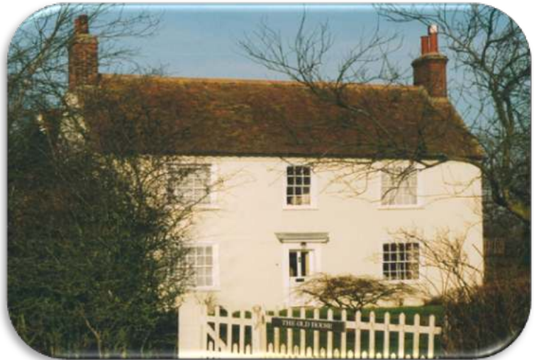
Original, small-pane vertical sliding sash windows
