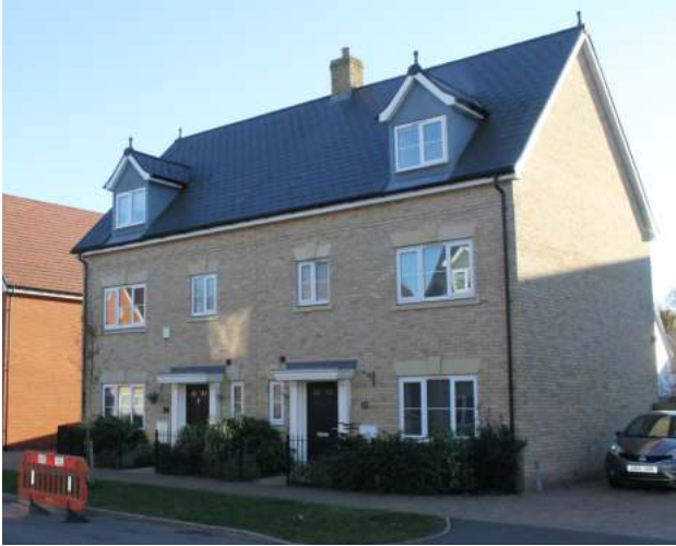
The design quality and Georgian style of this dwelling is undermined by the use of UPVC units (the juxtaposition between Georgian-style decorative stone lintel & plastic window is odd and stark)
