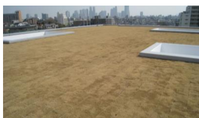
(10) Right after completion
