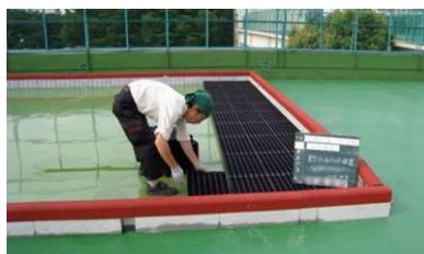
(2) Setting the water storage units
