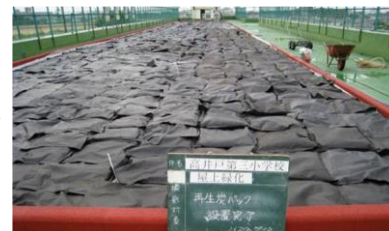
(6) Installation of the moisture holding regenerated charcoal bags
