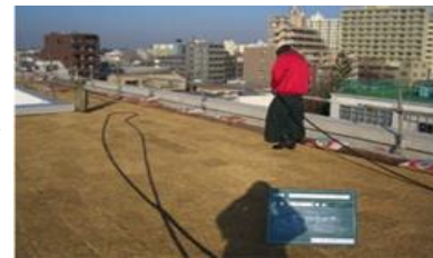
(9) Water after planting to ensure proper anchoring of the roots
