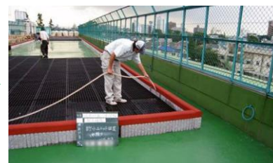
(3) Filling the water storage units
