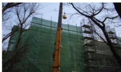
(1) Hoisting and unloading
