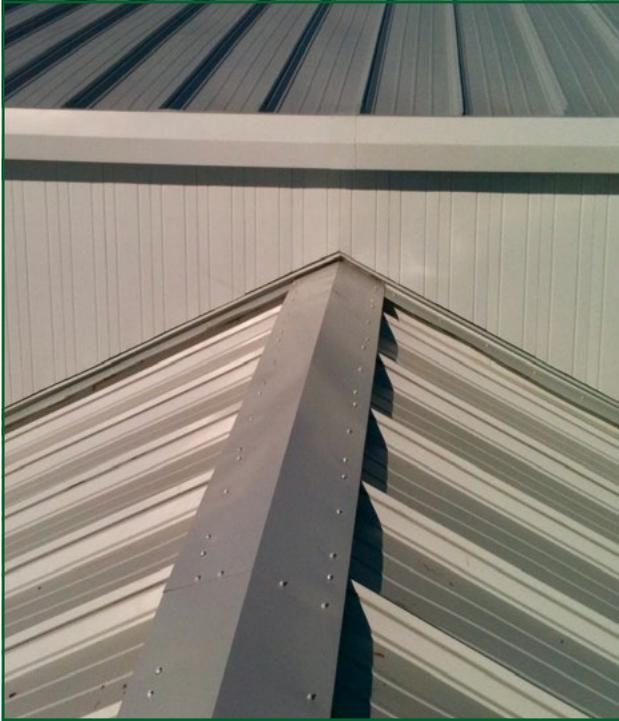
The TS-324™ Trapezoidal Panel is a structural metal roofing panel which provides superior wind and weather protection under all roof loading conditions. Typically installed over open framing, the trapezoidal profile maintains its structural integrity with a panel coverage of 24". The Trapezoidal Panel's ¼":12 minimum slope recommendation is the lowest of all metal roofing profiles offered by Union.
