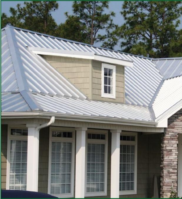
SL150 is a snap lock standing seam roof panel with 1.5" high ribs that installs with concealed clips. The clips allow the panel to freely expand and contract during thermal movement which can help ensure an aesthetically pleasing look when very long panel lengths are required. SL150 is popular in both residential and commercial applications and is a great choice for customers that prefer a taller rib profile or for roofs requiring very long panel lengths.
