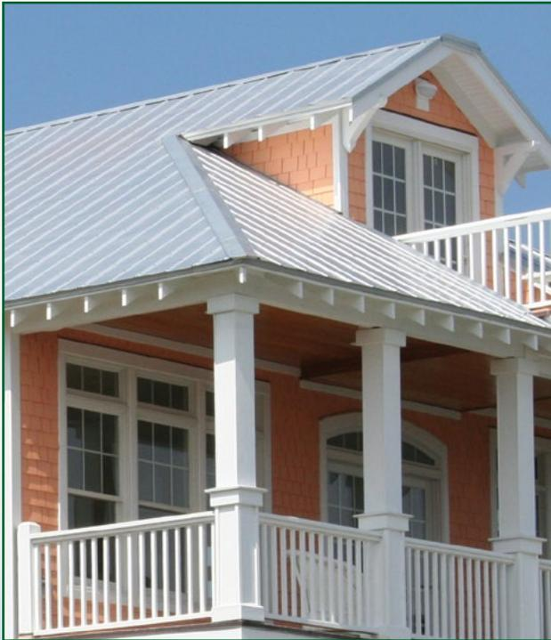
For generations, 5V metal roofing panels have been used on farm buildings and other rural metal roofing projects. Today, many homeowners have recognized that the timeless design is ideal for residential roofs as well. Our 5V metal roofing panels are especially popular in Florida and other coastal areas. Our 5V roof panels are designed with an enhanced “U” over “V” profile to provide maximum leak resistance.
