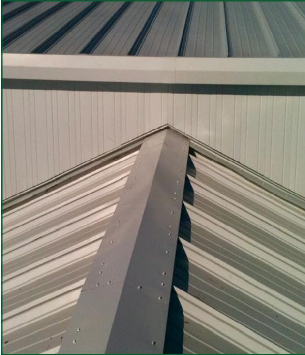
The TS-324™ Trapezoidal Panel is a structural metal roofing panel which provides superior wind and weather protection under all roof loading conditions. Typically installed over open framing, the trapezoidal profile maintains its structural integrity with a panel coverage of 24". The Trapezoidal Panel's 1/4":12 minimum slope recommendation is the lowest of all metal roofing profiles offered by Union.
