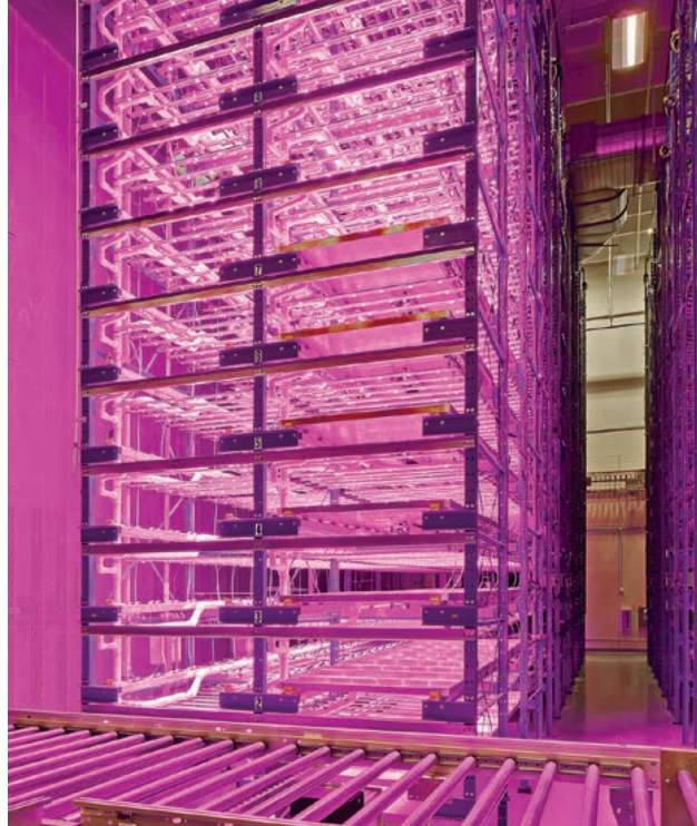
Higher environmental temperature uniformity is achieved with LED lights, at a much lower energy input. Lights are also low voltage and waterproof.
