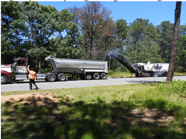
Grinder and Receiver Truck
