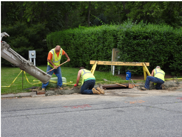
Highway Crew repairing curbing and drainage basin.
