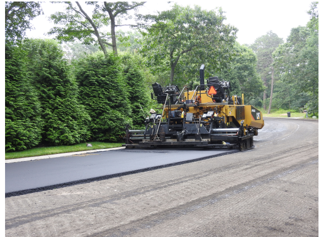
Asphalt Paver at Work
