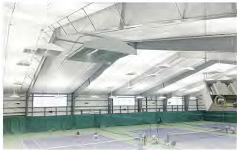
Fort Collins Country Club - Large Building Trusses Affected LED Light Distribution
