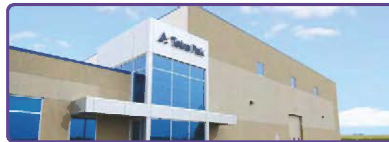
EXAMPLE: PRE-CAST BUILDING INVESTS HEAVILY IN THE FRONT ENTRY AND UNIFORMLY AROUND THE ENTIRE FACADE
