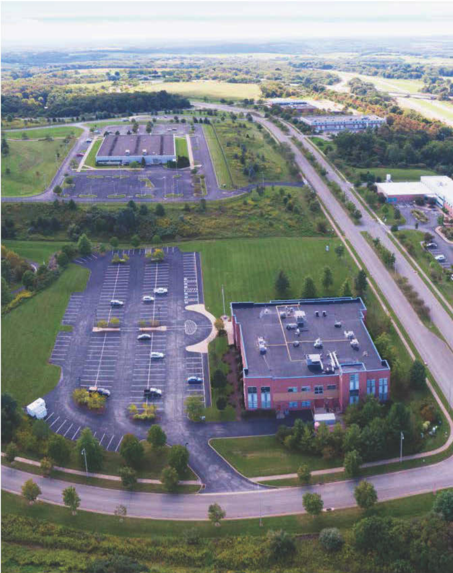
Northpointe Industrial Park's screening and landscaping in Freeport, PA
