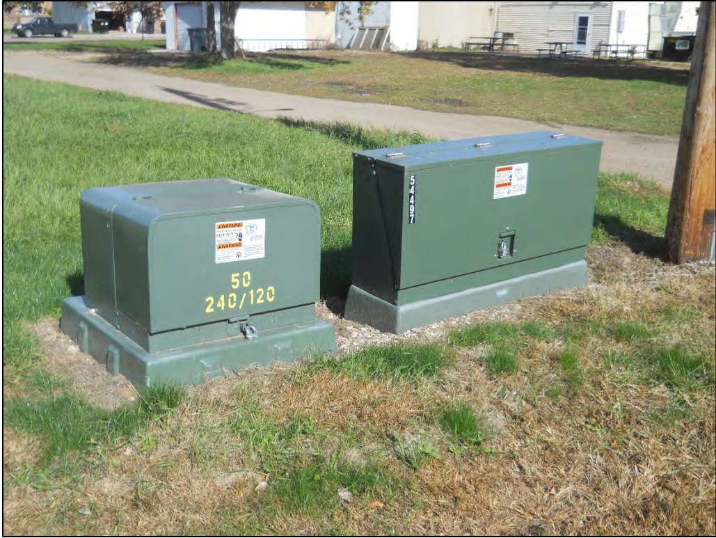
Electrical transformer and box across alley to west of site.
