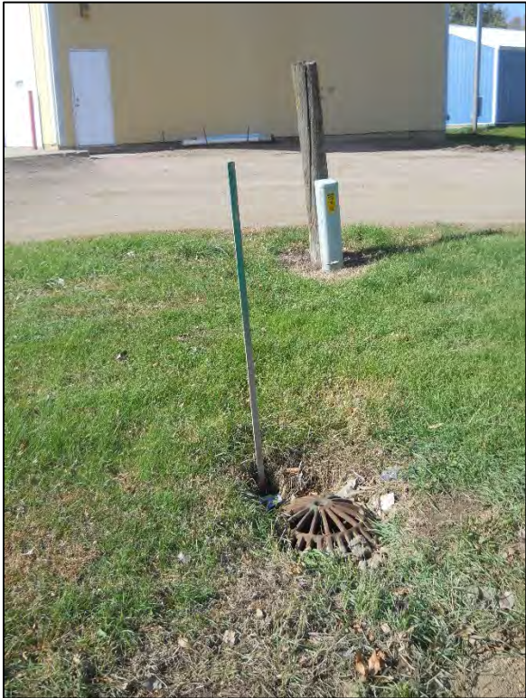
Storm sewer catch basin near southwest corner of site.
