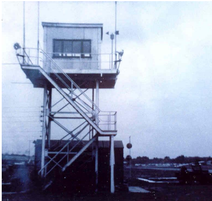
The Control Tower.
