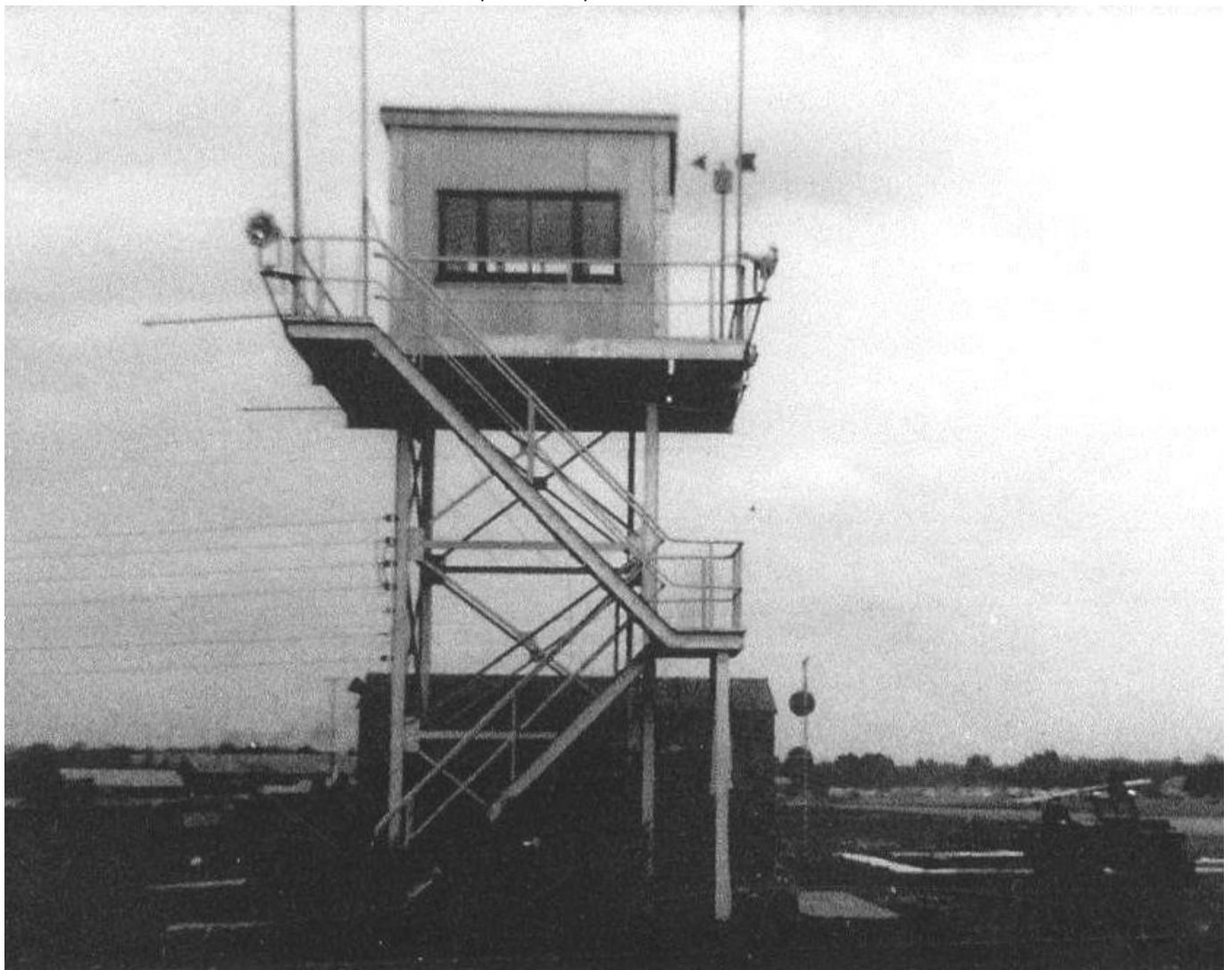
Christchurch Control tower.
