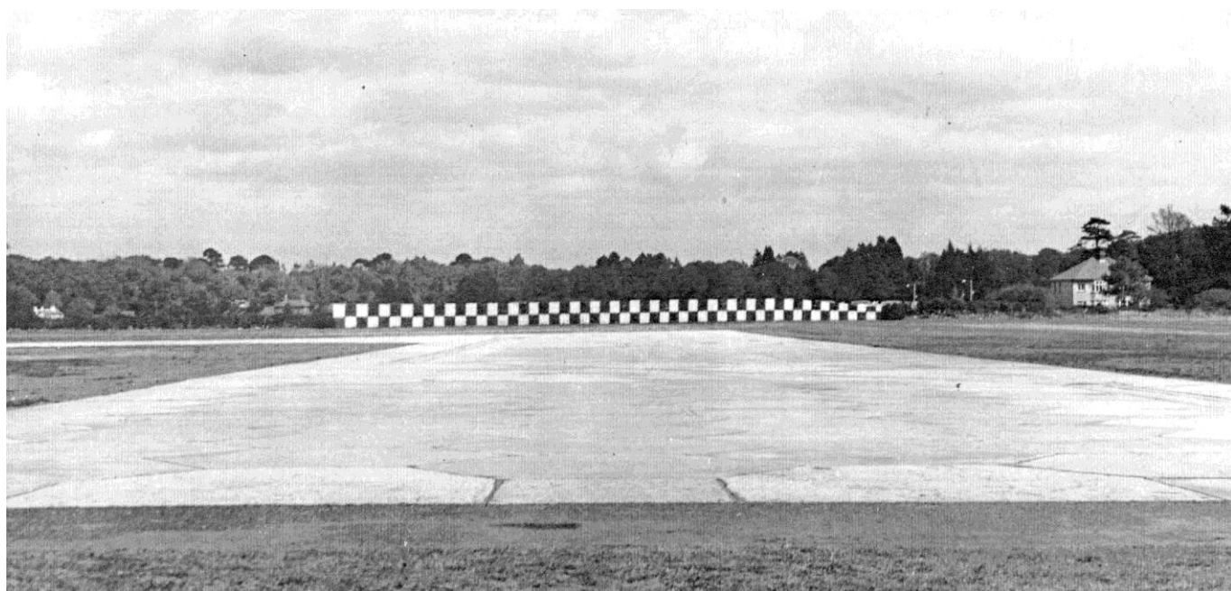
Photo taken at the eastern end of the main runway (later concreted by MEXE). Looking at the runway end. Lymington Road is beyond the checkerboard markers. The run-up area and holding point is to the left.
