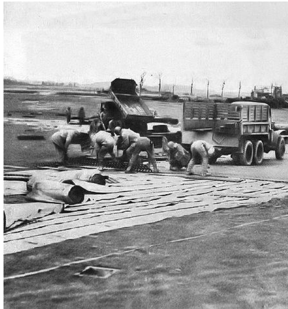
Prefabricated Hessian Runway being Laid. Picture from US National Archives
