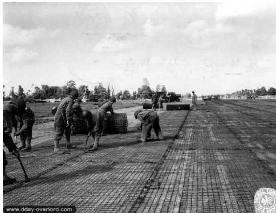
Square Mesh Tracking Runway being Laid. Picture from US National Archives
