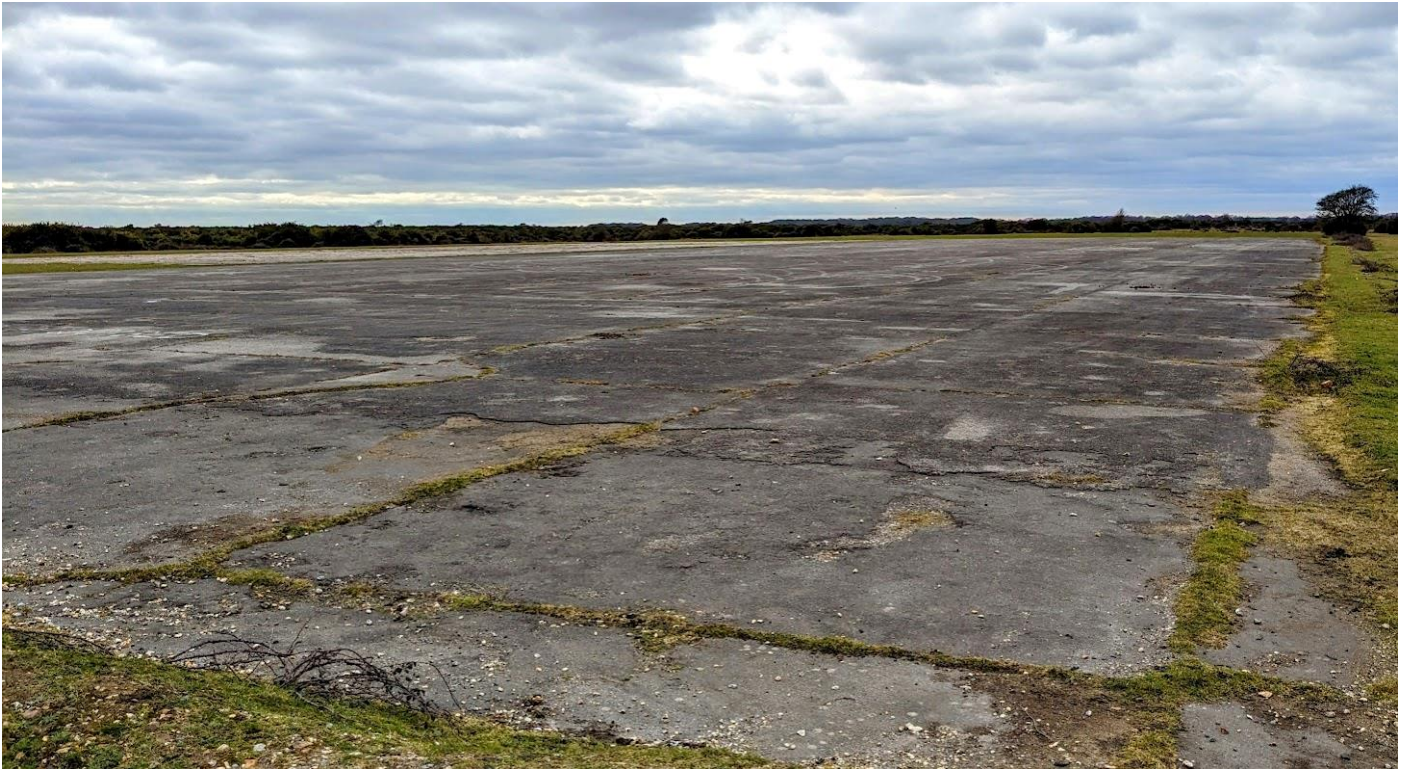
The remains of the start of runway 34 at RAF Beaulieu
