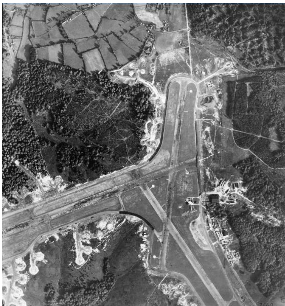
Aerial photograph of the east end of Stoney Cross airfield looking north, the control tower, airfield code and technical site are to the right (copyright @iwm.org.uk)
