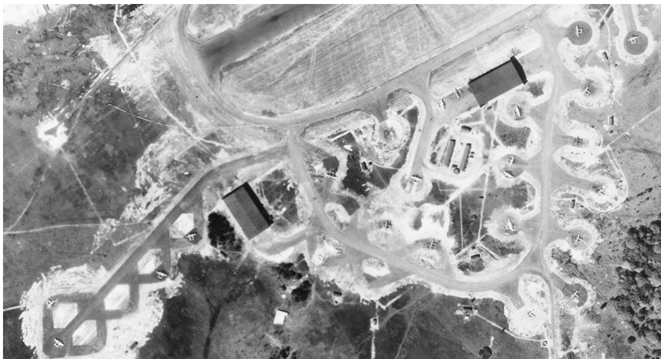
Stoney Cross airfield looking north on April 30, 1944 (copyright@iwm.org.uk)
