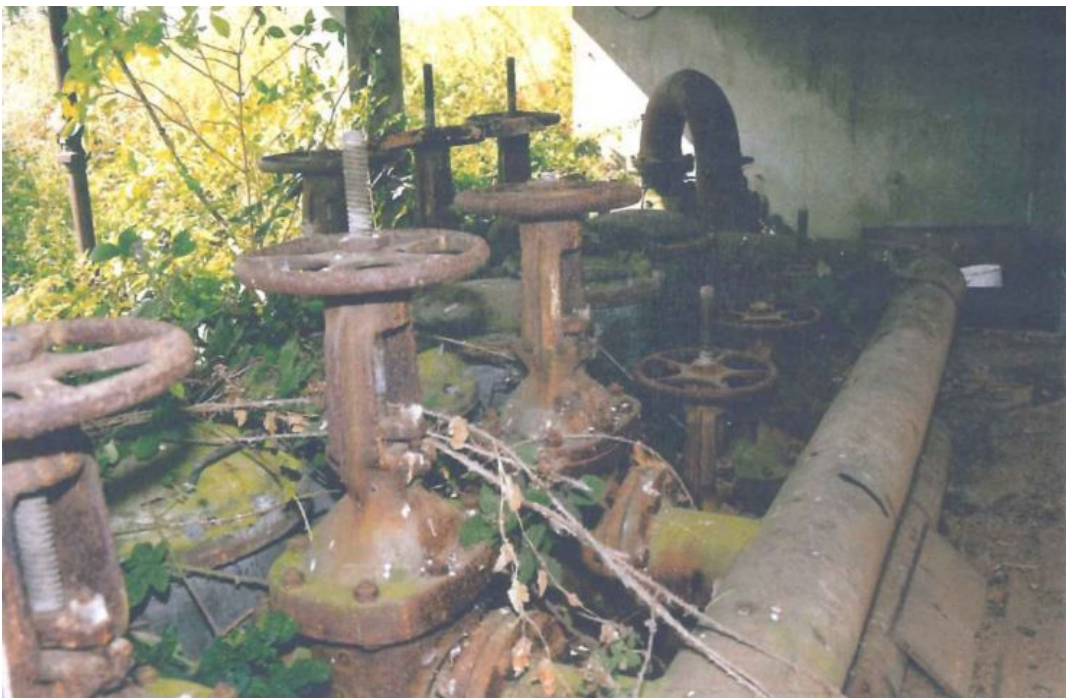
The 2 pictures above shoes the POL (Petrol, Oil and Lubricant in Clastres. It was used to bring the aviation gas up to the hardstands (Eddie Rosier/archives 367 th FG)
