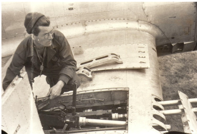
Armorer of the 393rd FS installing or removing one of the machine gun of a P-47 of the unit. The eight 0.5 caliber machine guns of the P-47 could send a terrific amount of lead to against the enemy targets (archives 367 th FG)
