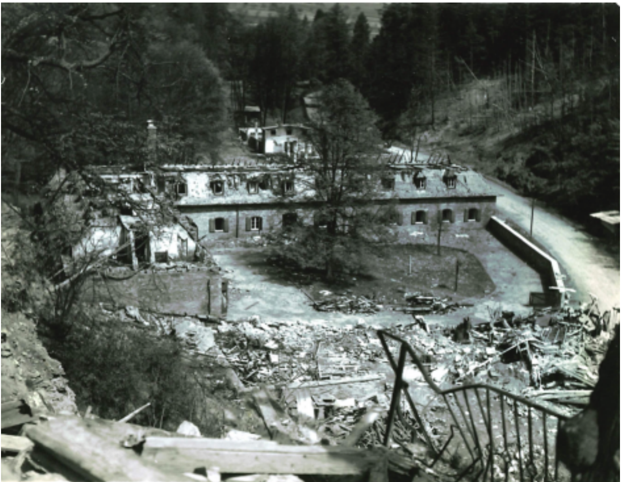
Wreck of the castle of Ziegenberg after the attack by the P-47 Thunderbolt of the 367 th FG. This is the front view of the L shaped building (archives 367 th FG)
