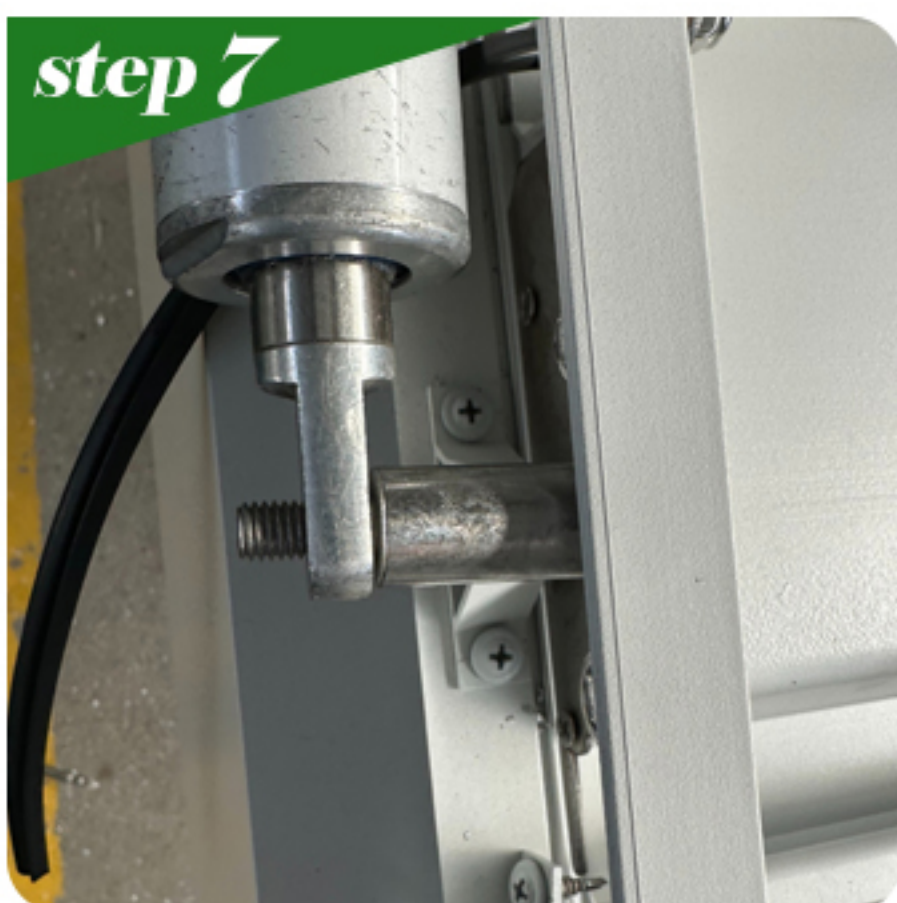
Fix the motor, thread the bolts, and tighten the screws (1 washer facing inward and 2 washers facing outward)
