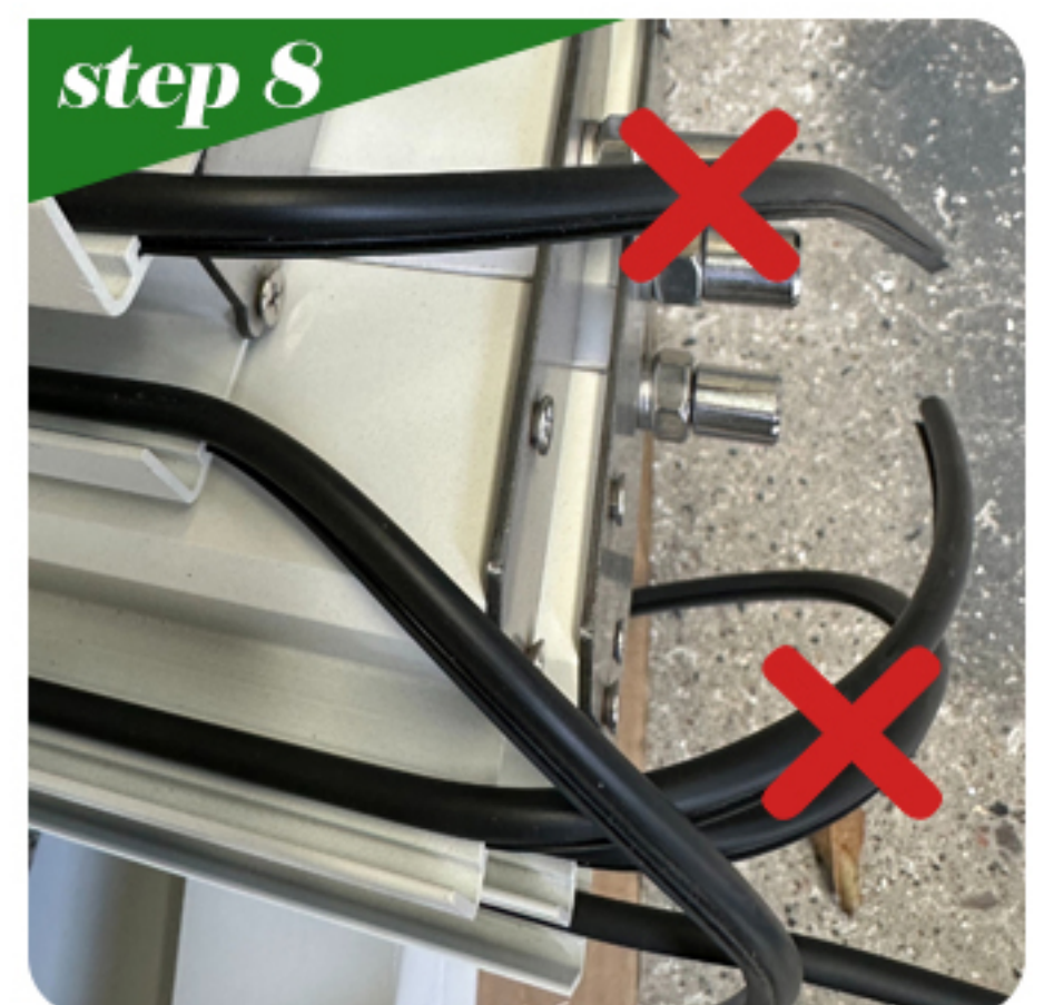
Wiring, cut off excess waterproof strips, and install them
