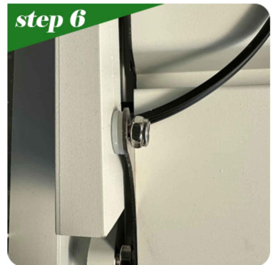
Thread the motor push rod, connect the blades, and tighten the screws
