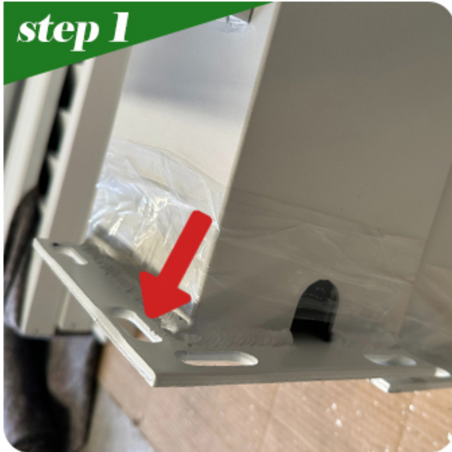
Install screws on the ground and install vertical columns
