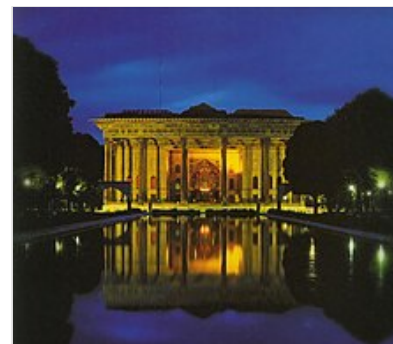
Chehel Sotoun Palace in Isfahan , built during the 17th century with example of a talar , UNESCO World Heritage Site . [627]
