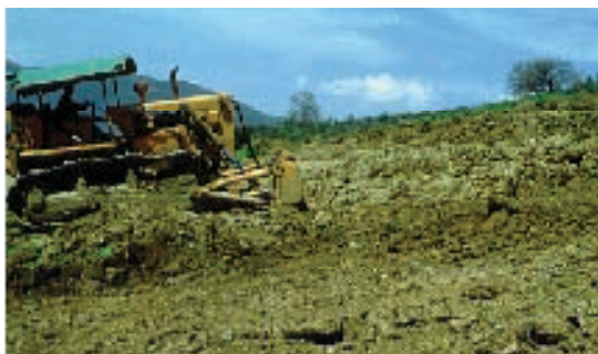
Figure 20. Levelling the site.
