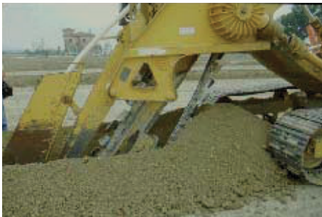
Figure 23. Digging and laying drainage pipes.
