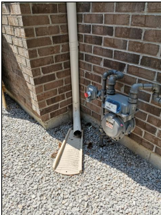
11. Should discharge 6 feet from building
