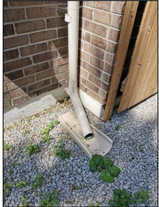
10. Should discharge 6 feet from building
