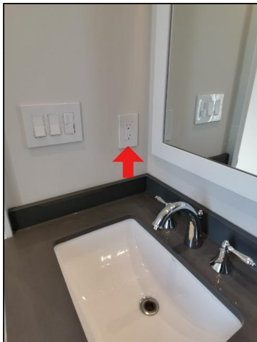
35. GFCI/GFI needed (Ground Fault Circuit...
