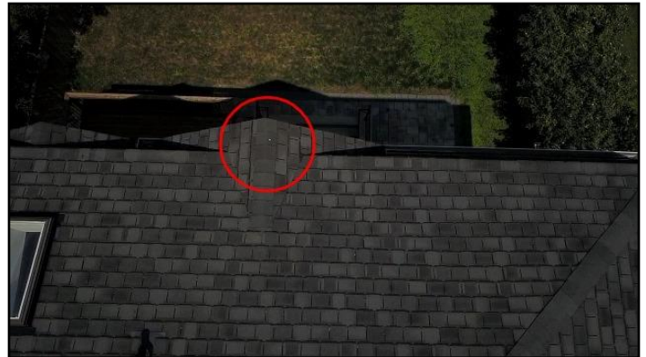
2. Exposed fasteners
