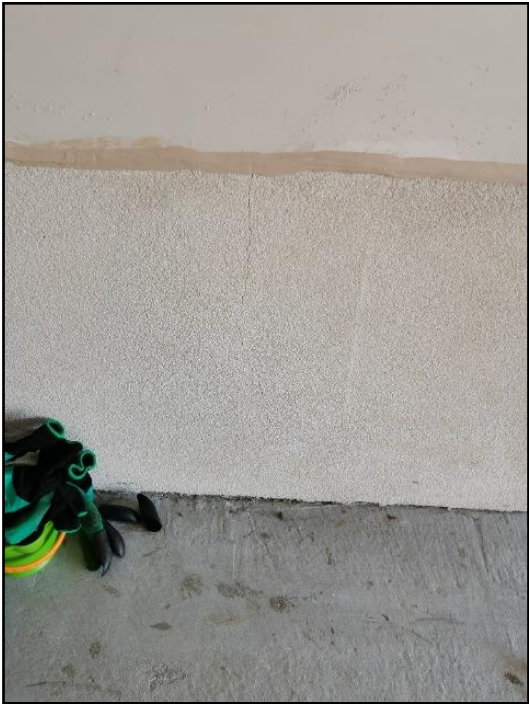
25. Typical minor cracks
