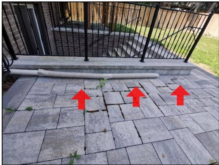
18. Slope toward building
