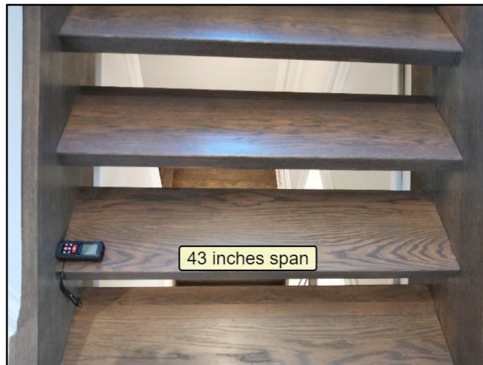
66. Excessive span between stringers
