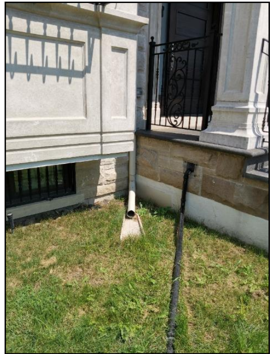
8. Should discharge 6 feet from building
