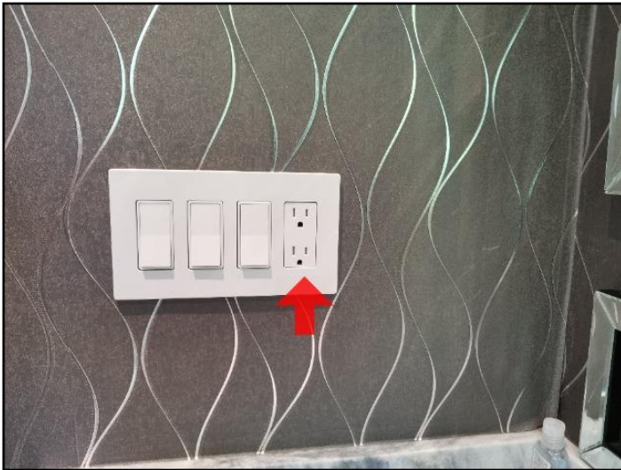
33. GFCI/GFI needed (Ground Fault Circuit...
