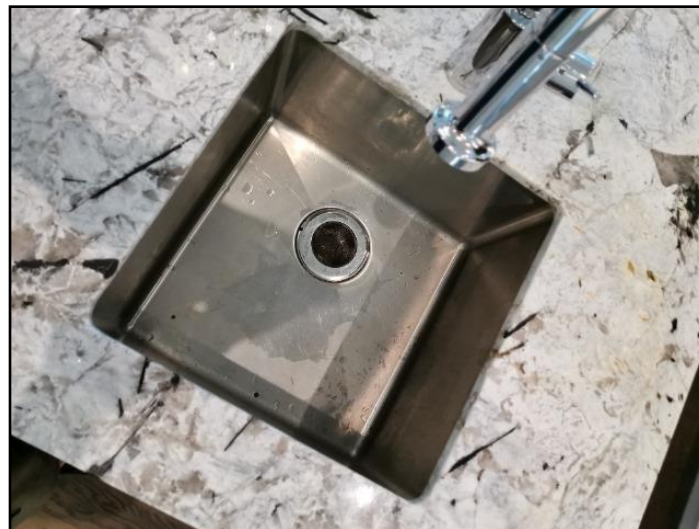
47. Overflows missing, leak, rust or...
