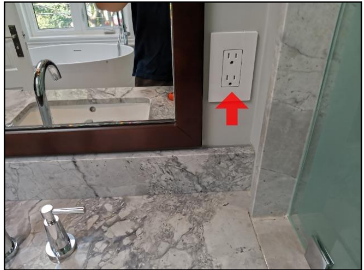
34. GFCI/GFI needed (Ground Fault Circuit...
