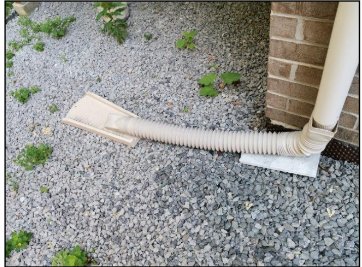
14. Should discharge 6 feet from building
