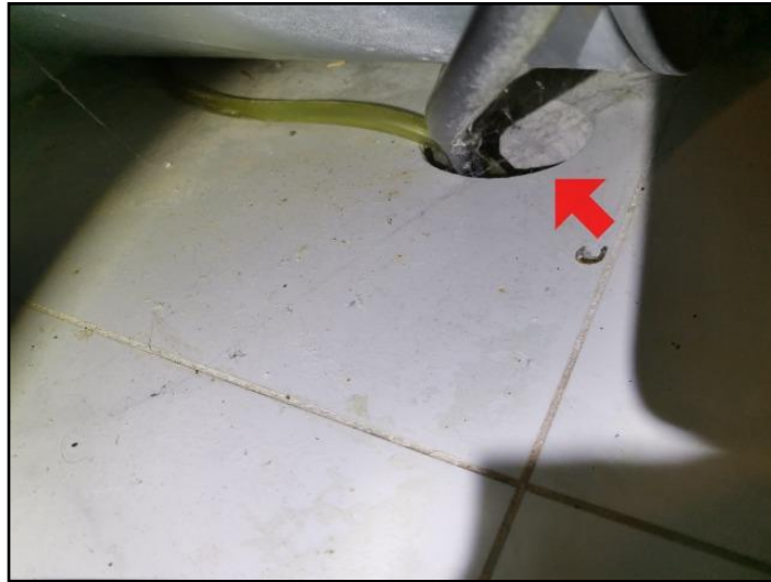
42. Grate missing, rusted or obstructed
