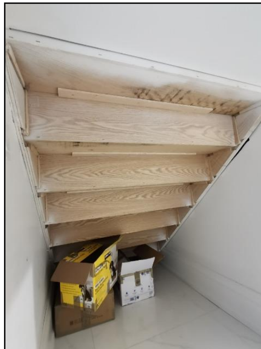
65. Drywall missing or incomplete on underside...
