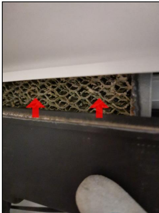
39. Clogged pad, mesh or nozzle
