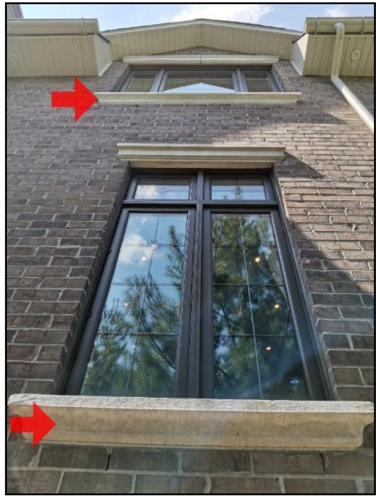
16. No capillary break (drip edge) on sill
