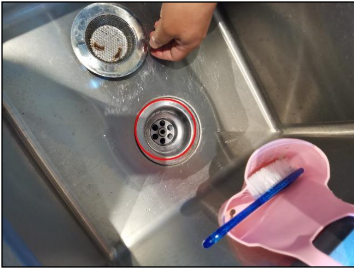
48. Drain stop missing
