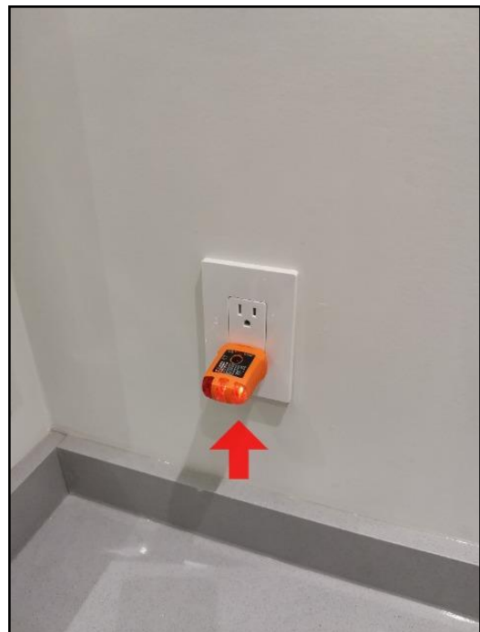
36. GFCI/GFI needed (Ground Fault Circuit...
