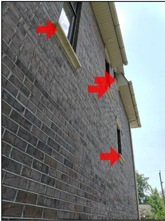
15. No capillary break (drip edge) on sill
