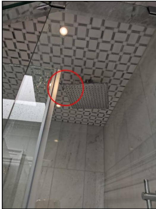
45. Shower head damaged
