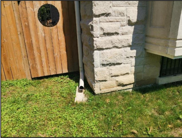
9. Should discharge 6 feet from building
