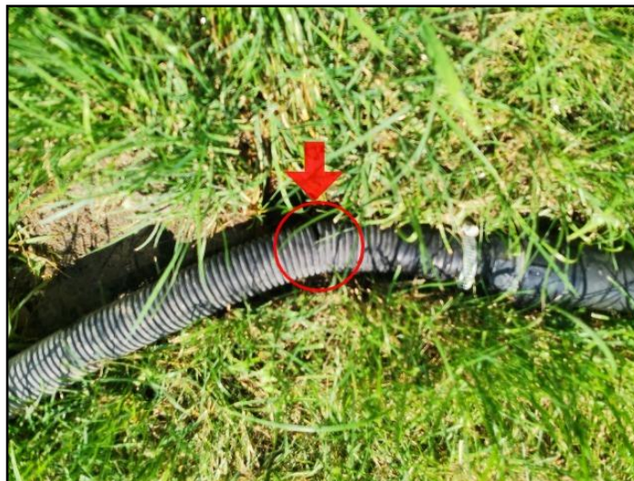
43. Discharge pipe problems
