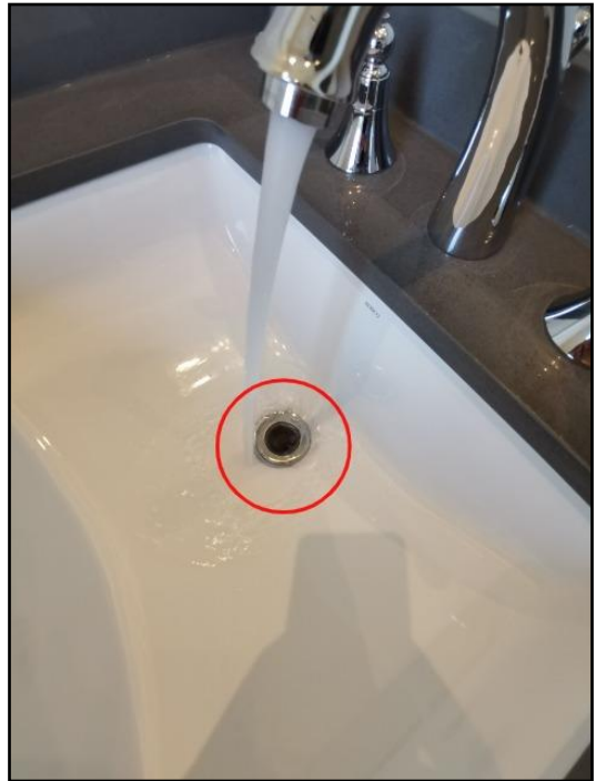
49. Drain stop missing
