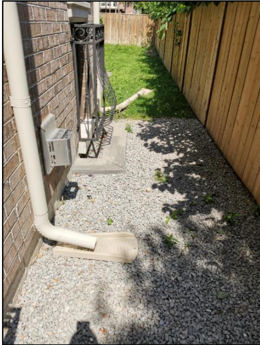
13. Should discharge 6 feet from building
