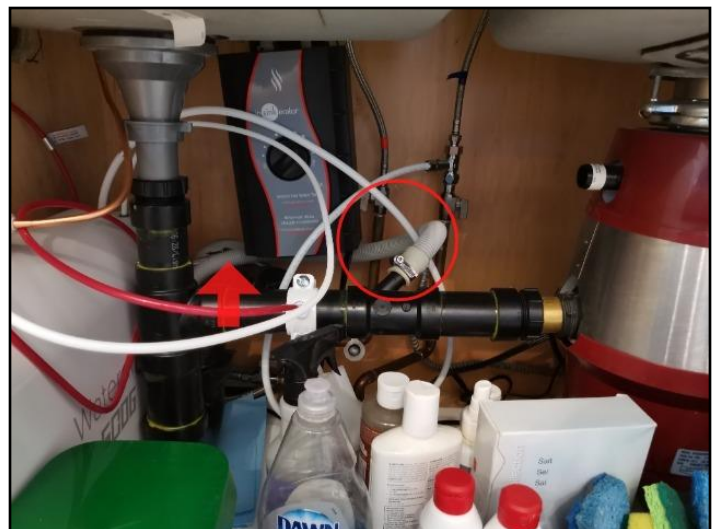
176. Backflow prevention high loop missing
