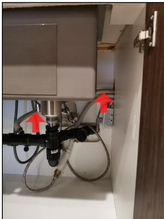
175. Backflow prevention high loop missing
