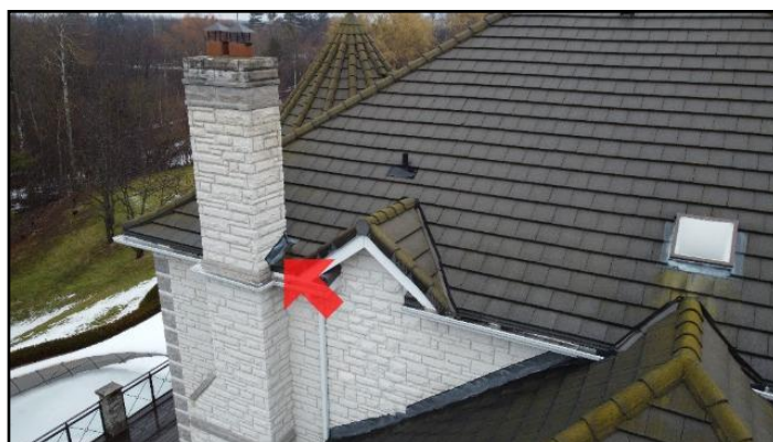
13. Not let into mortar joints
