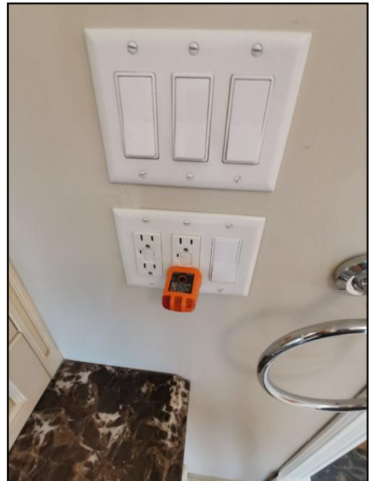
80. Test faulty on GFCI/GFI (Ground Fault...
