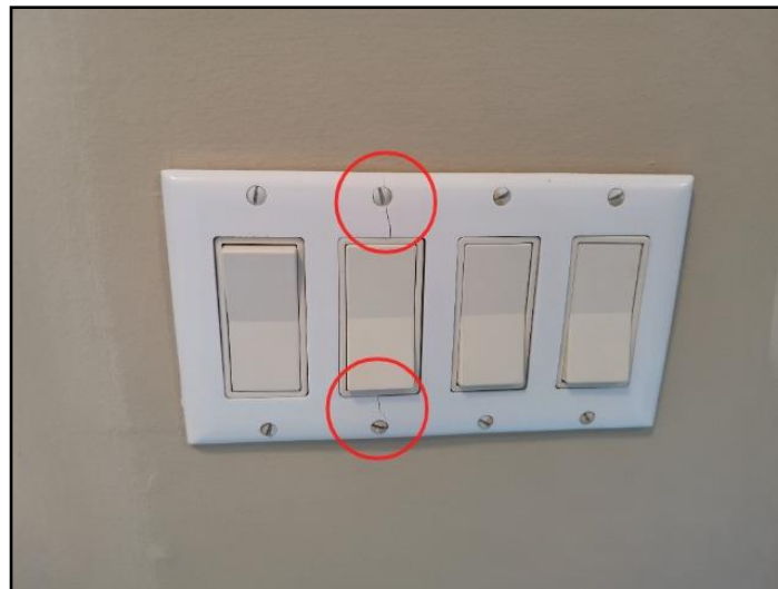
83. For switch is damaged
