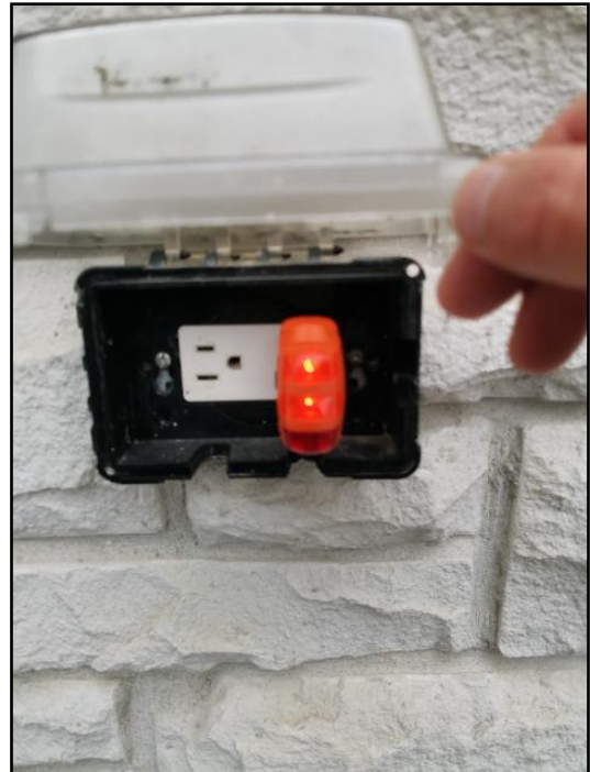
73. Not suitable for outdoor (exterior) use
