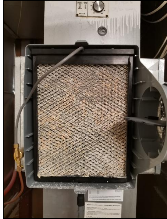
102. Clogged pad, mesh or nozzle
