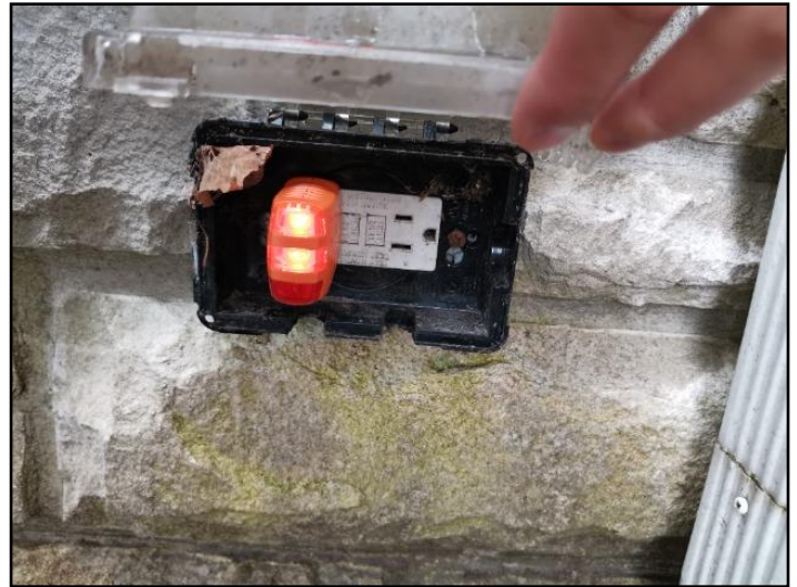
78. Test faulty on GFCI/GFI (Ground Fault...
