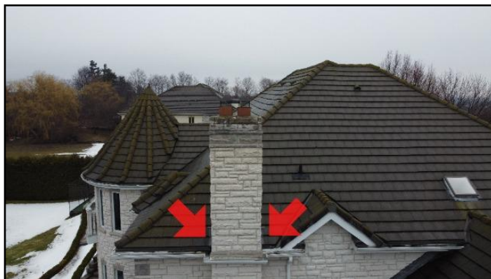
14. Side flashings not set into shingles properly
