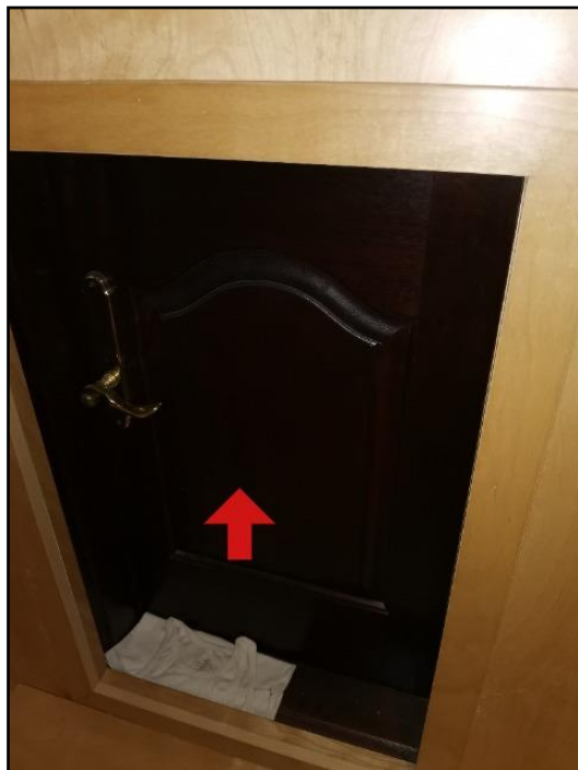
112. Not insulated and not weatherstripped
