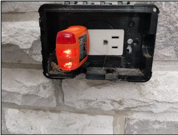
74. Not suitable for outdoor (exterior) use
