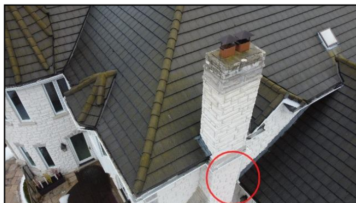
20. Kickout flashing - missing
