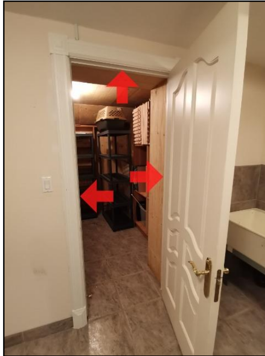
168. Weatherstripping missing around door
