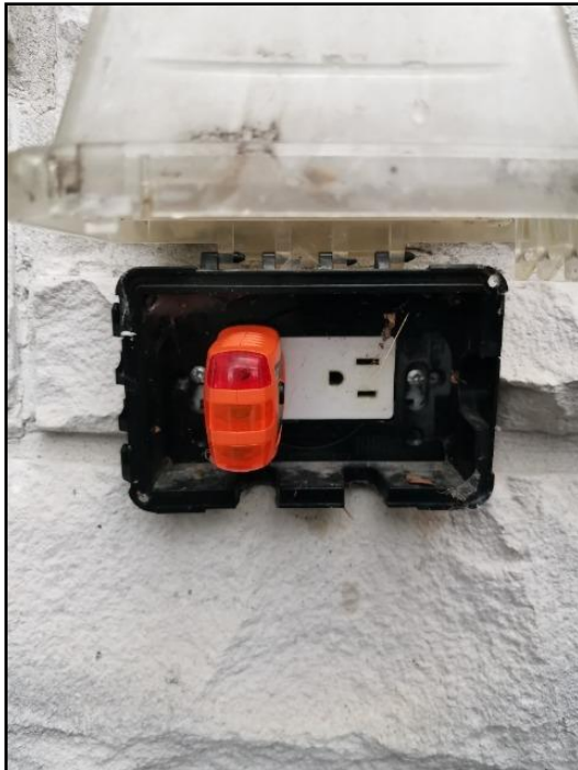
72. Not suitable for outdoor (exterior) use
