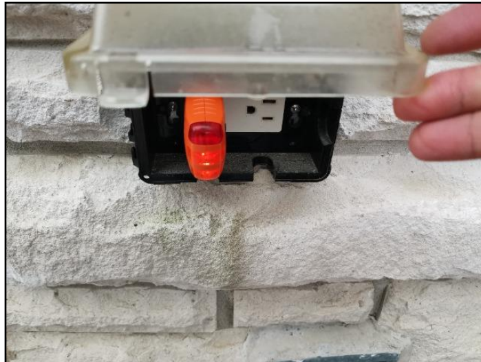
76. Not suitable for outdoor (exterior) use
