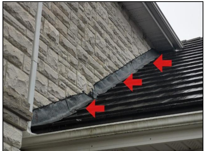
17. Step flashings not set into shingles properly
