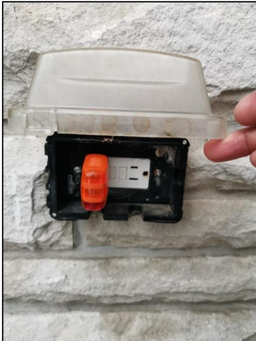
77. Test faulty on GFCI/GFI (Ground Fault...
