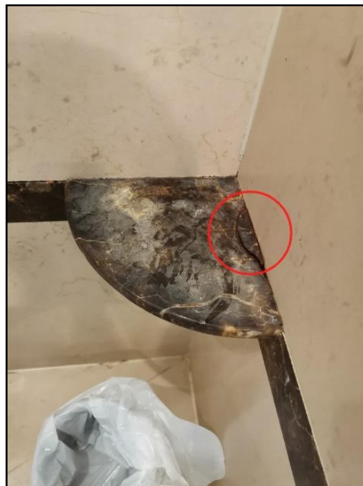
163. Tiles loose, missing, cracked, stained or...
