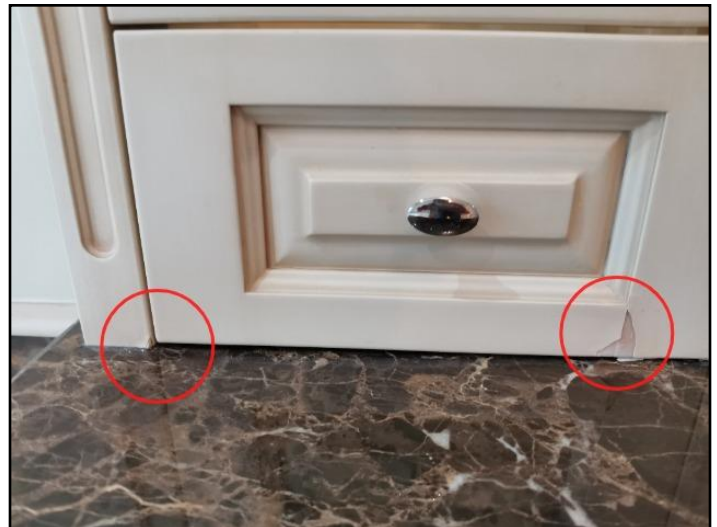
160. Water damage
