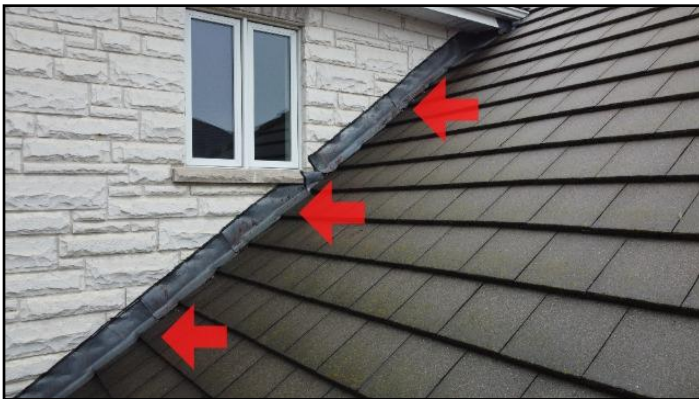
16. Step flashings not set into shingles properly
