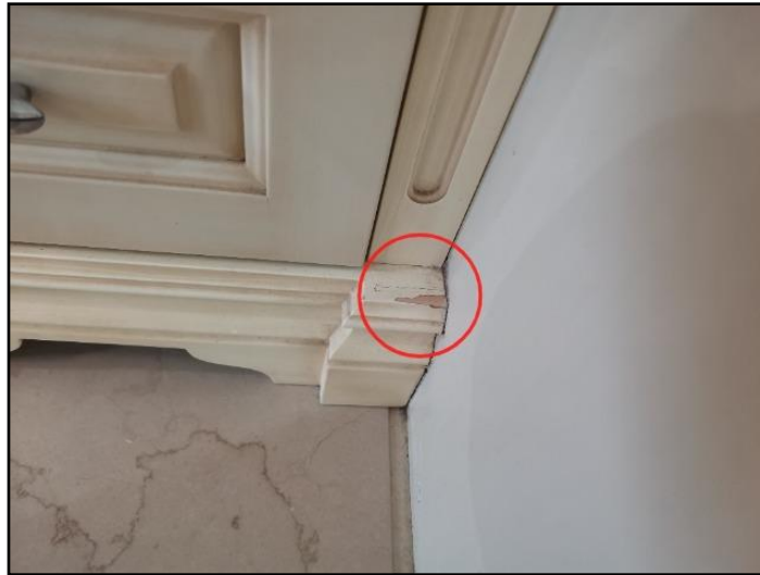
161. Water damage
