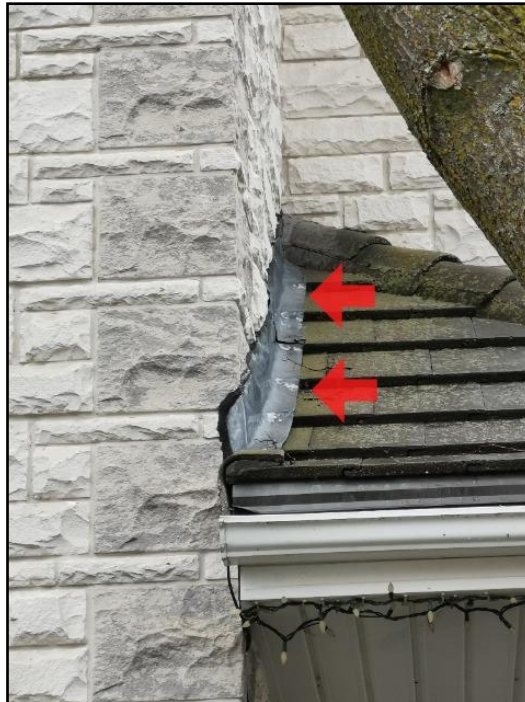
18. Step flashings not set into shingles properly
