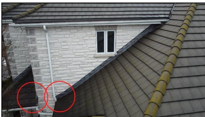
19. Kickout flashing - missing
