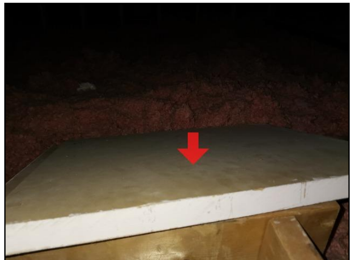
113. Not insulated and not weatherstripped
