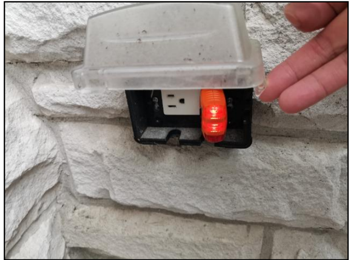
75. Not suitable for outdoor (exterior) use
