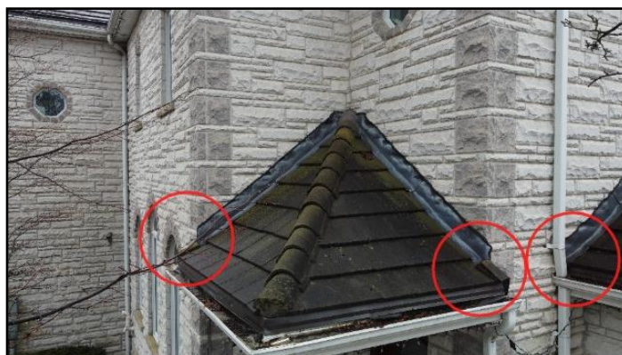
21. Kickout flashing - missing
