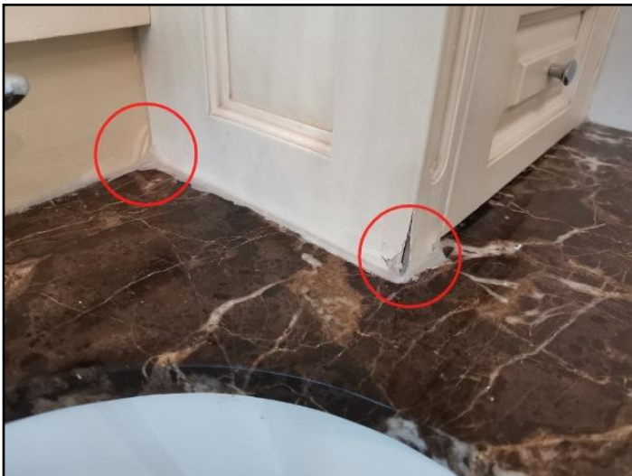
159. Water damage
