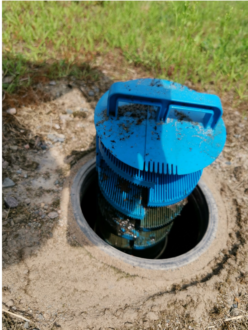
Figure 4: Effluent filter
