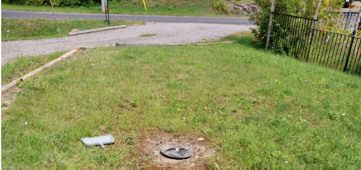
Figure 6: Leaching Field (South looking North)
