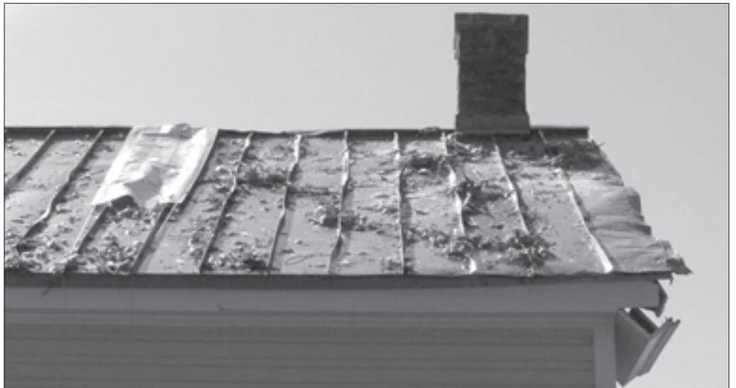
*When the branches were removed, the damage to the roof's east side became visible.*
