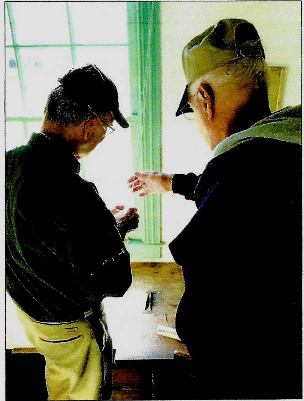
Volunteers Jeff Klapper and Jack Fringer, along with Carol Khalili (not shown), installed six new ultraviolet-light-blocking roller blinds.
