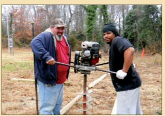
Workmen dug post holes for the new split-rail fence marking the old road.
